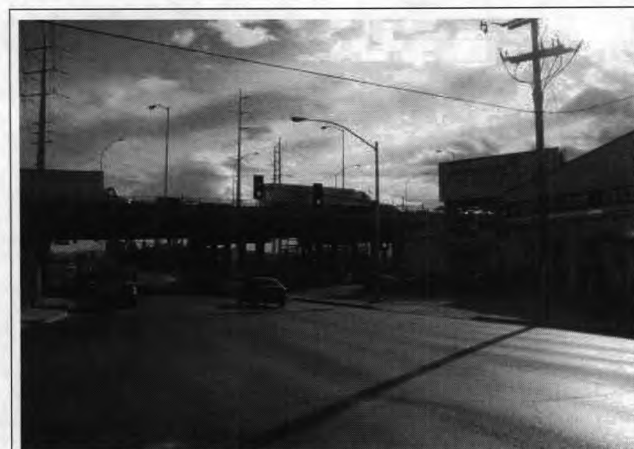
Closer look at the Sahara Avenue overpass.
