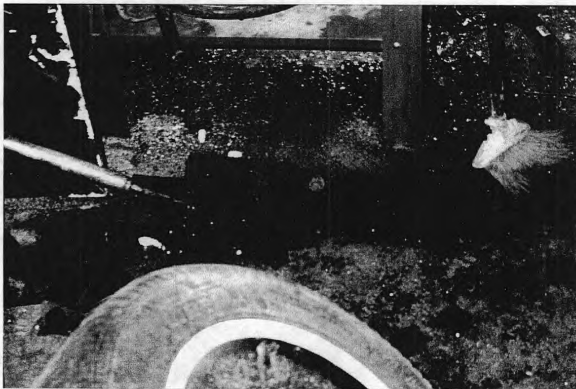
Photo #16: View of the stained floor below the degreasing station along the north wall.
