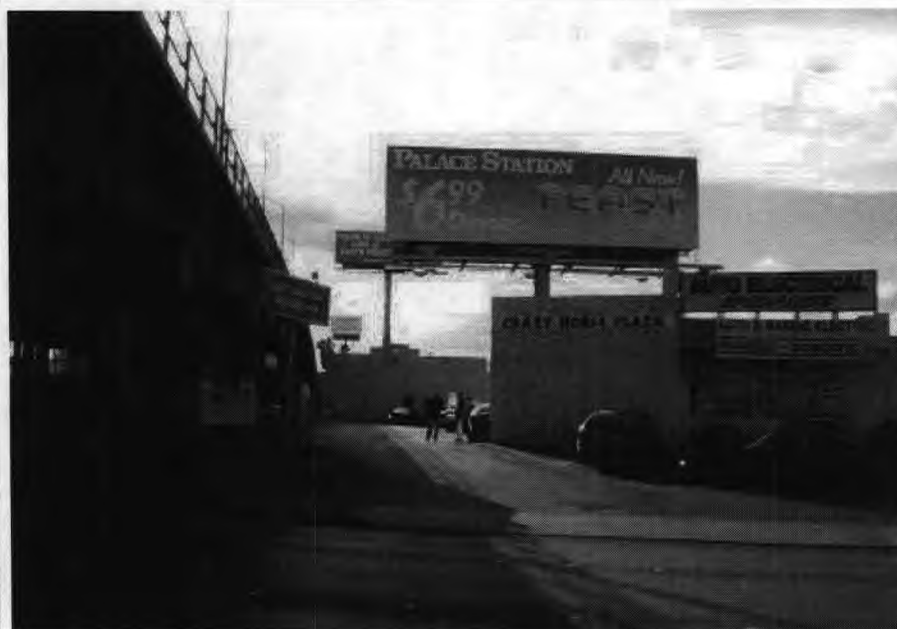
Looking west at south end of subject. Note subject billboard.
