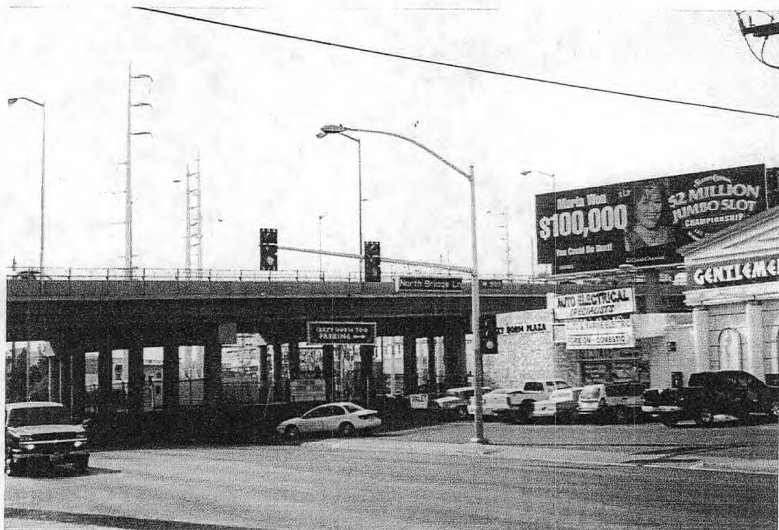
Photo #4: View of the elevated section of Sahara Avenue that runs along the south boundary of the Crazy Horse Plaza Property.
