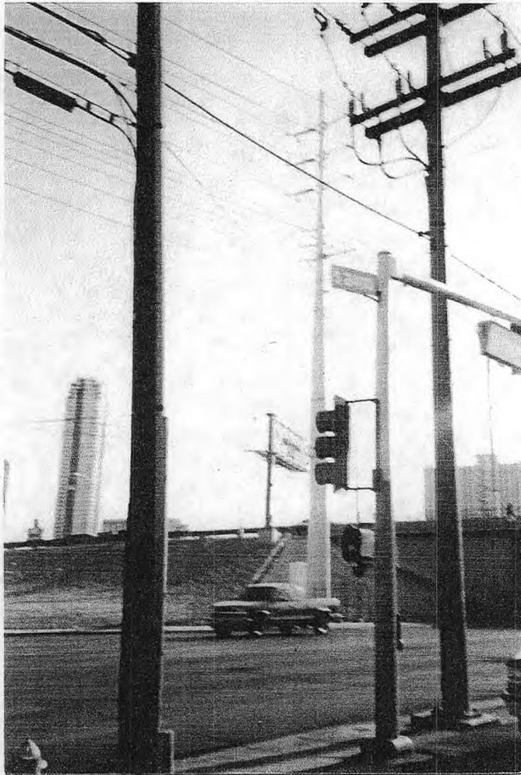
Photo #11: View of the high voltage electrical transmission lines running along the east side of Industrial Road. Lower voltage distribution lines run along the west side of the street.
