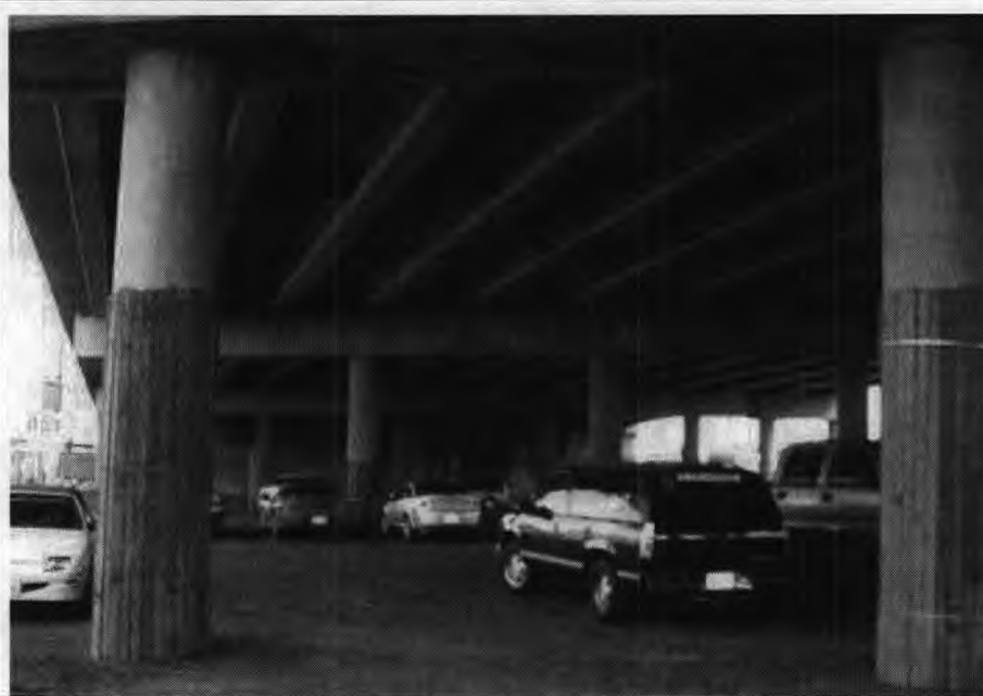
View of leased land to the south used for parking under Sahara.
