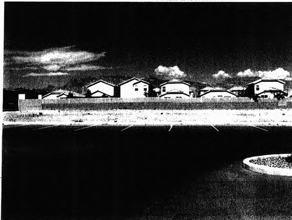
WEST VIEW BEFORE T-MOBILE INSTALLATION
