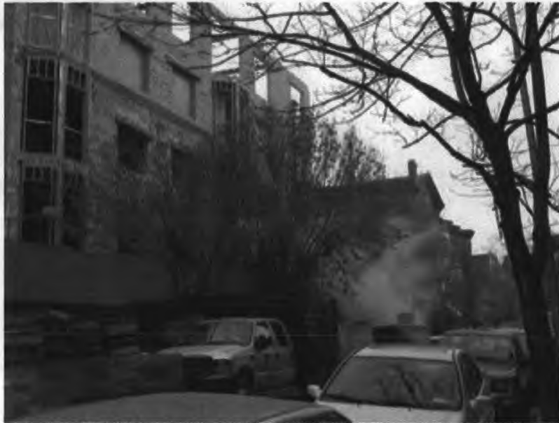
December 15, 2005 - smoke from the construction happening at the corner of Sterling and Seventh Ave., the site of the 1960 crash.
