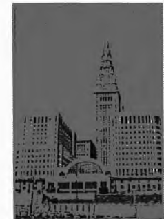
Tower City Center, Cleveland
