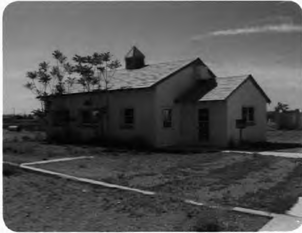
Generator Building and Swimming Pool. The generator building was constructed to supply power to the ranch and make it a self-sufficient operation. The swimming pool, currently filled in, was one of the later comforts that Goumond added to the ranch to appeal to his paying clientele.
