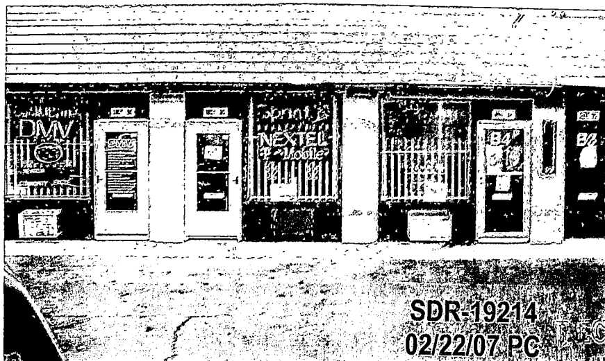
BLD B B3-5 FACING SOUTH
