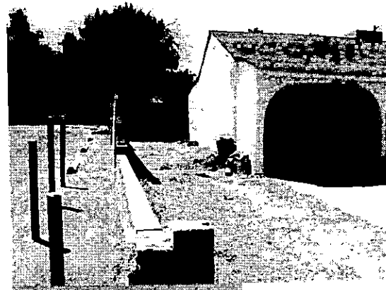
DRIVEWAY SIDE - SOUTH
