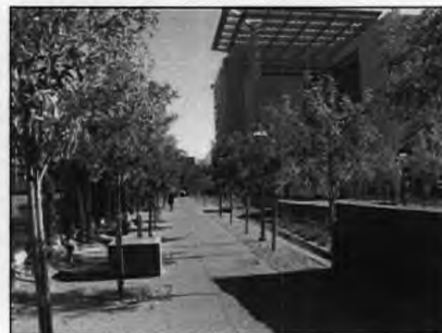
PHOTO 10: LEWIS AVENUE IMPROVEMENTS
