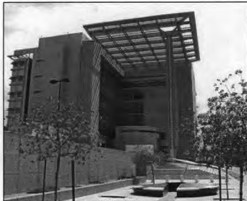
PHOTO 6: FEDERAL BUILDING / U.S. COURTHOUSE
