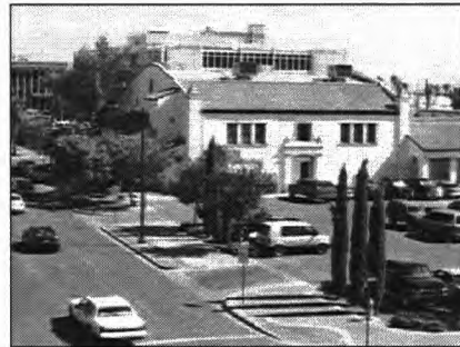
PHOTO 8: FOURTH STREET CORRIDOR IMPROVEMENTS
