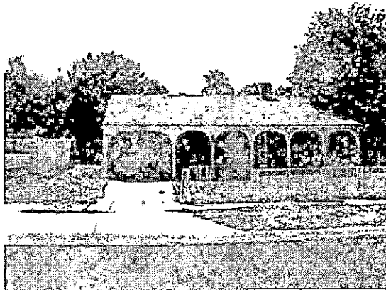
FRONT OF BUILDING - EAST
