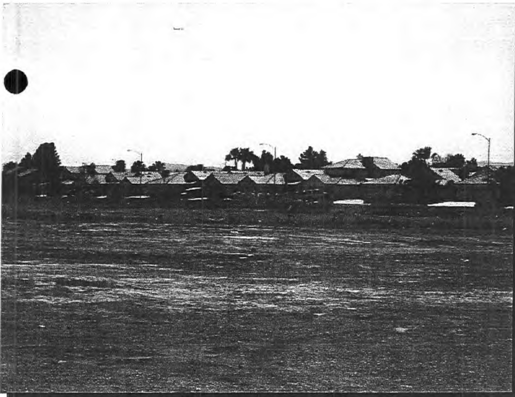
Northeast border on Harris Avenue looking southwest.
