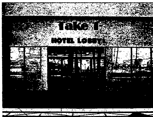
Side Entrance Signage
