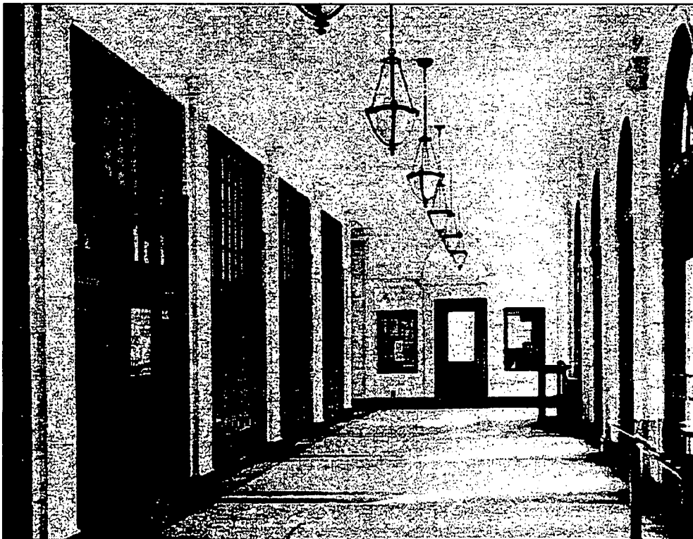
Figure 6: Post Office Lobby, view east, 1933 (General Services Administration, Slide Number NV000536, Building Number NV0005ZZ)
