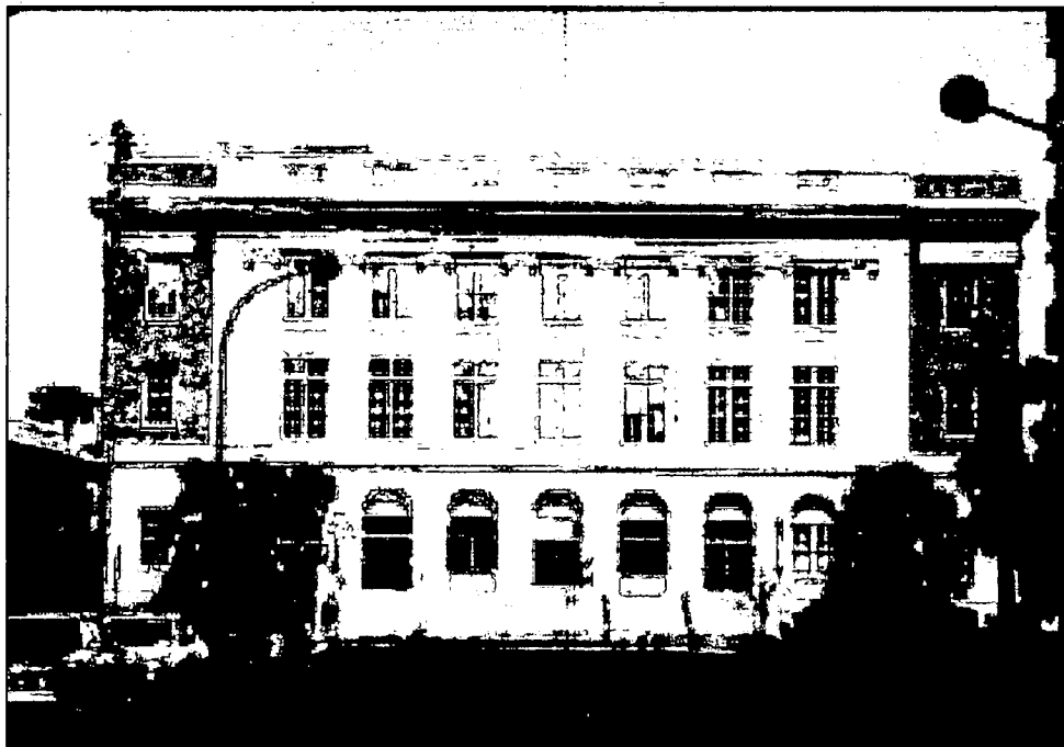
Figure 16: Las Vegas United States Post Office and Courthouse, view north (c.1980)
