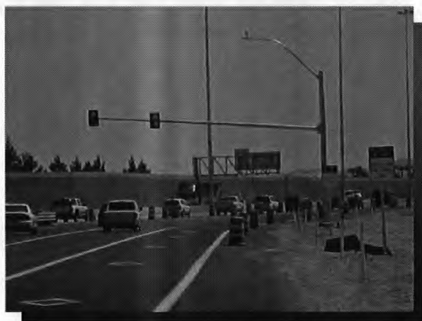
Ramp meters at Southbound US-95 and Cheyenne
