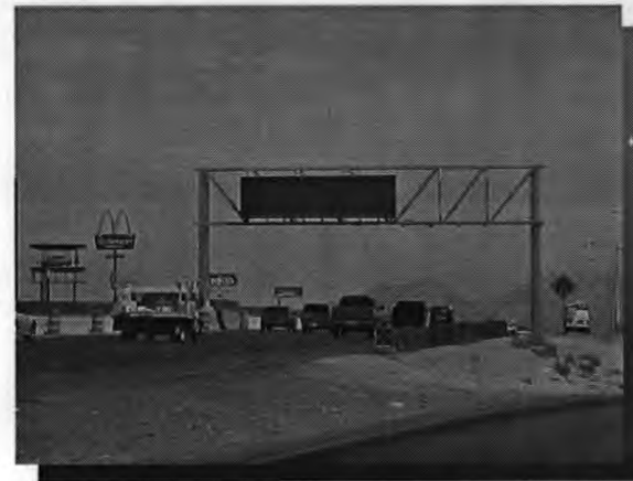
Southbound US-95 north of Jones Blvd.
