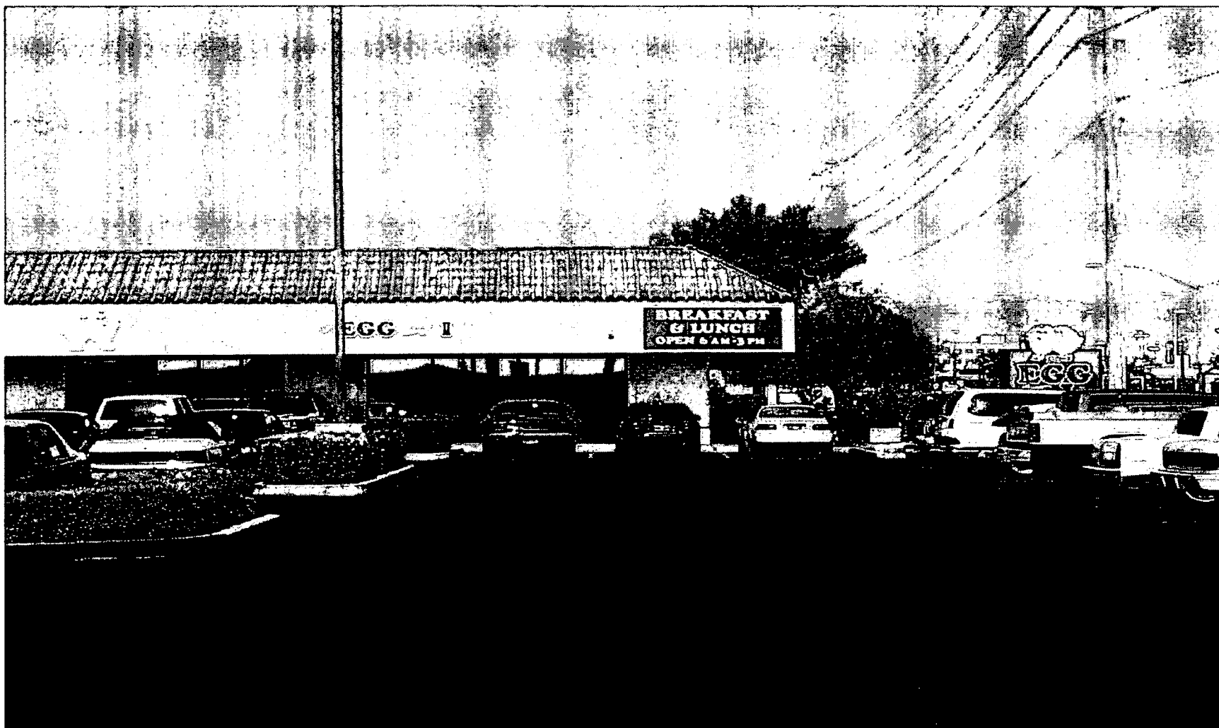
U-0071-00 - FROM EAST SIDE OF SITE LOOKING WESTERLY TO EXISTING RESTAURANT (SAHARA AVENUE IS AT RIGHT)
