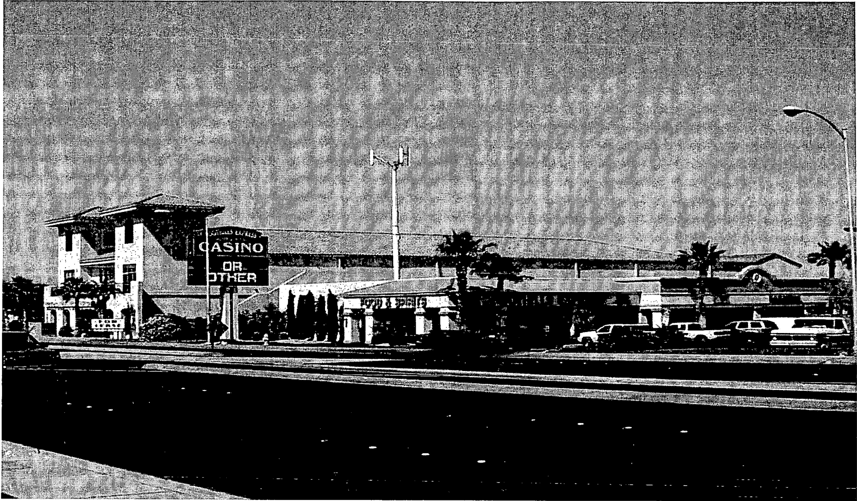
U-0067-00 - FROM SOUTHWEST OF SITE LOOKING NORTHEASTERLY TO EXISTING MONOPOLE (RAINBOW BOULEVARD SEEN IN FOREGROUND)
