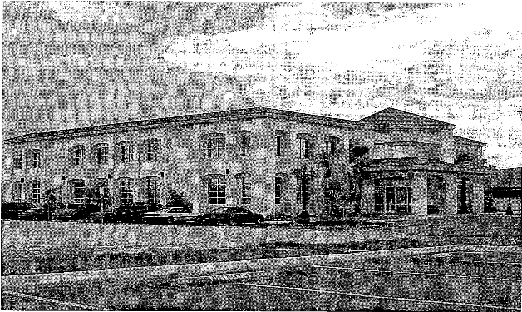
U-92-99 - from the northwestern corner of the site.
