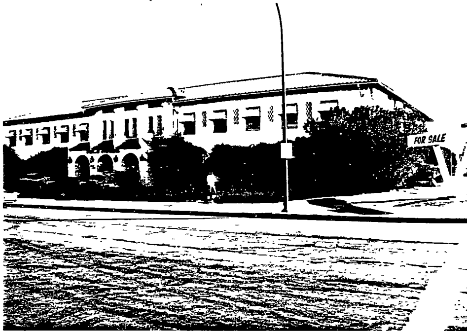
(3) Oslo House, corner of 8th and Ogden. Former "flop-house", building is now closed. Building has been vacant for over a year.
