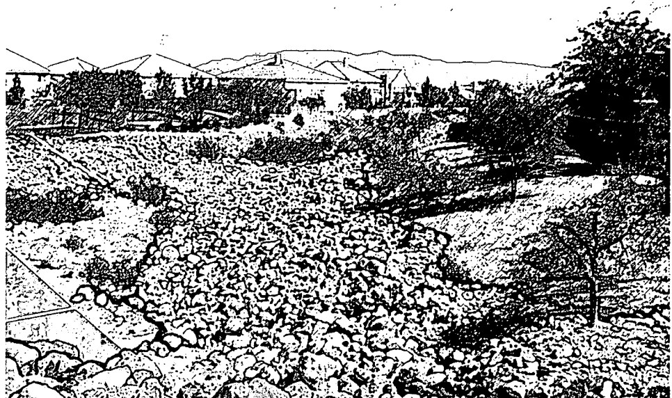
An example of the preferred use of natural materials in flood channel design.
