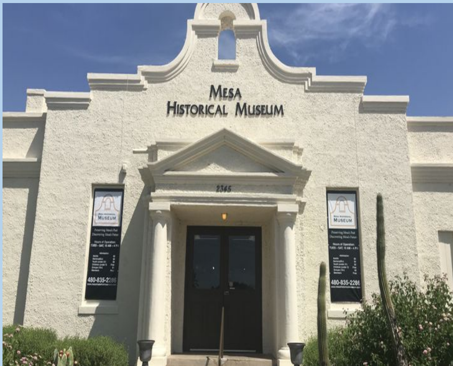
Mesa, AZ Renovated 1914 four-room schoolhouse
