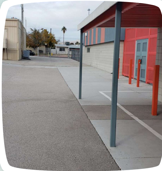
Exterior of school
