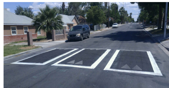
EXAMPLE SPEED CUSHION LAYOUT ON 15TH STREET
