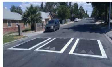
EXAMPLE SPEED CUSHION LAYOUT ON 15TH STREET
