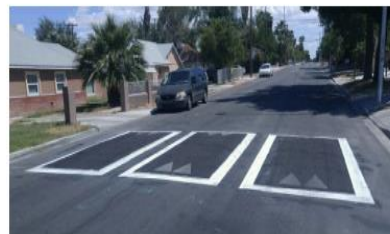
EXAMPLE SPEED CUSHION LAYOUT ON 15TH STREET
