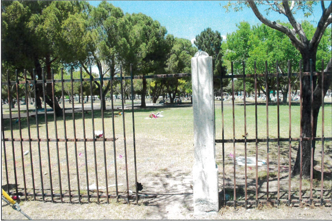
Image 5: Deteriorated and damaged fence.
