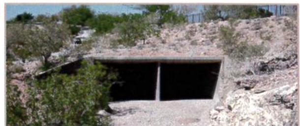
Figure 5. (2), 18' x 12' RCB inlet under Hualapai Way, looking northeast (downstream). Angel Park Golf Course is immediately to the north (left).
