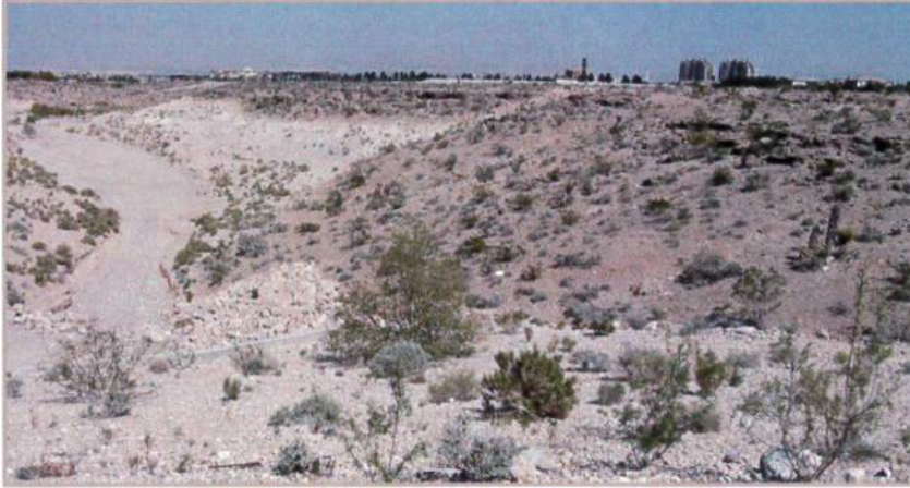
Figure 3. View of channel looking east from Hualapai Way. Note the caliche at the top of the channel. The bottom and sides appear graded, comprised of sand and gravel.
