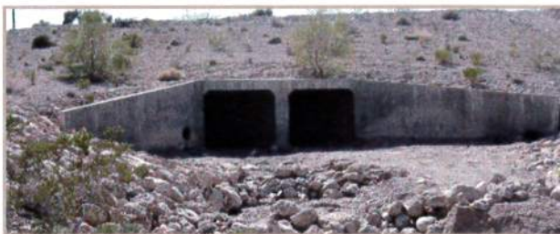
Figure 4. (2), 12' x 10' RCB outlet under Hualapai Way, looking west (upstream). Note 24-inch outlet on south wingwall.
