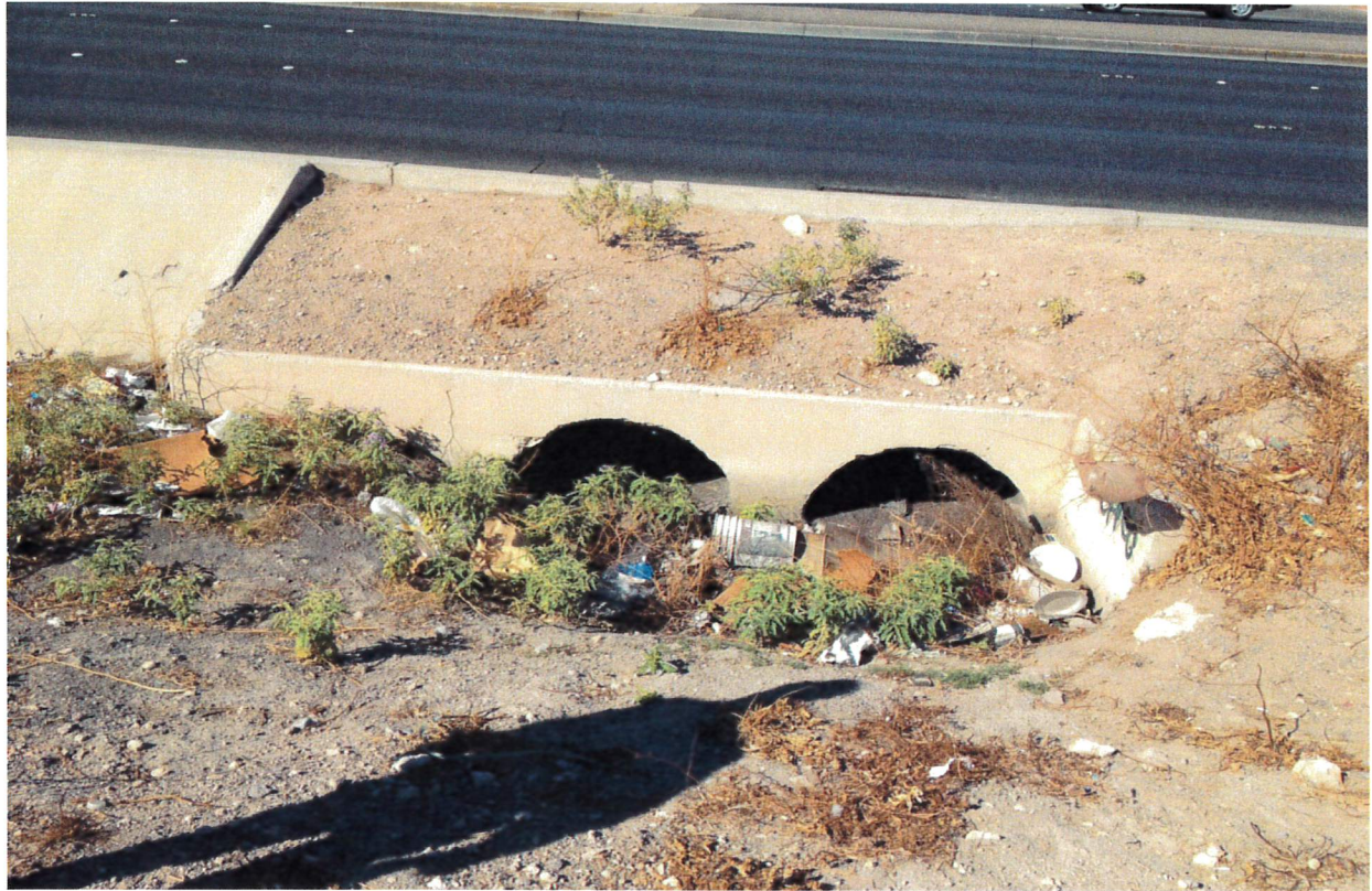
Approximate Station "L" 65+00 , on East Side of Rancho Drive: Two existing 43-inch x 27-inch CMP's
