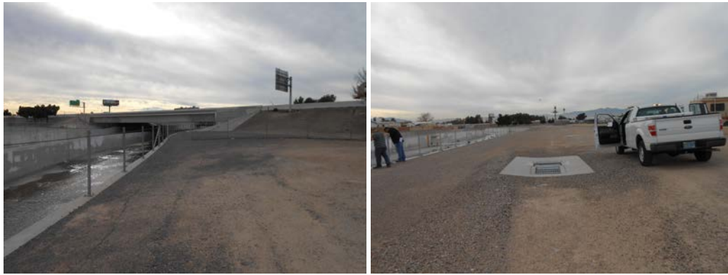
Image 16: Flamingo Wash Flood Control Channel north side looking west (left) Flamingo Wash Flood Control Channel north side looking west with storm drain drop inlet (right)
