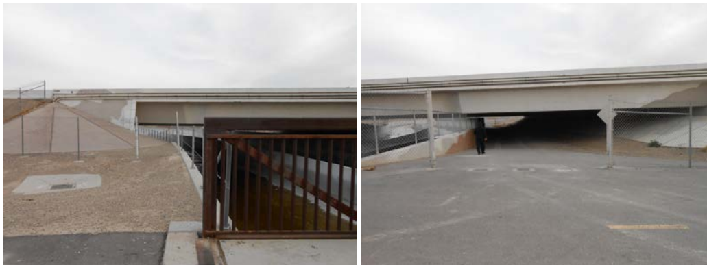
Image 15: Flamingo Wash Flood Control Channel north side looking east at Flamingo Arroyo Trail (left) Flamingo Wash Flood Control Channel south side looking east at Flamingo Arroyo Trail (right)
