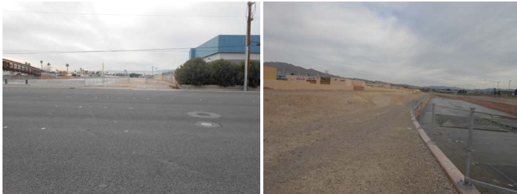
Image 17: Flamingo Wash Flood Control Channel north side looking west at Lamb Blvd (left) Flamingo Wash Flood Control Channel north side looking east at Lamb Blvd (right)
