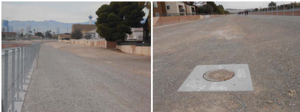
Image 18: Flamingo Wash Flood Control Channel north side looking west (left) Flamingo Wash Flood Control Channel north side looking east (right)
