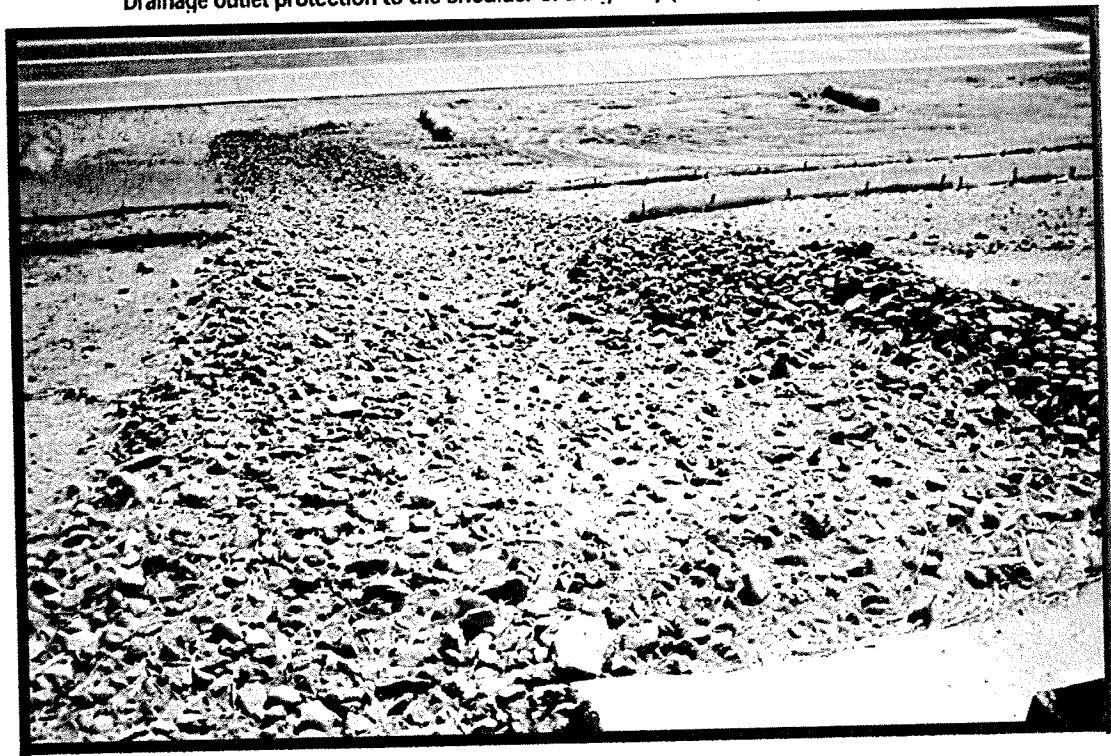
Drainage outlet protection to the shoulder of a highway (Courtesy of Maricopa County)
