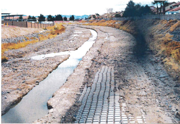
Las Vegas Wash on top of Bonanza Bridge looking south. Note cable-concrete block lining over sanitary sewer.
