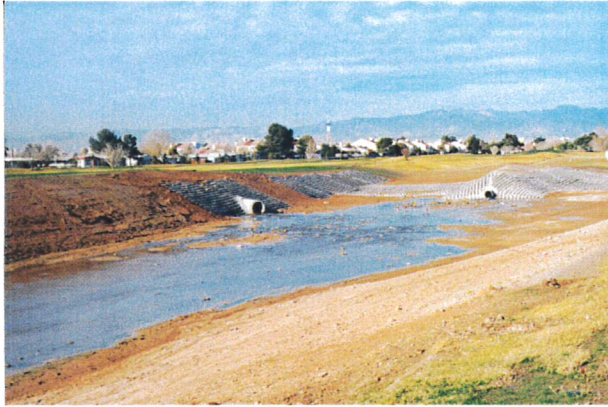
Las Vegas Wash and Flamingo Wash confluence after installation of cable-concrete block lining.
