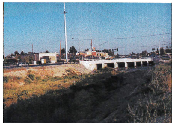
South of Lake Mead Boulevard looking north at culverts and proposed access ramp location.
