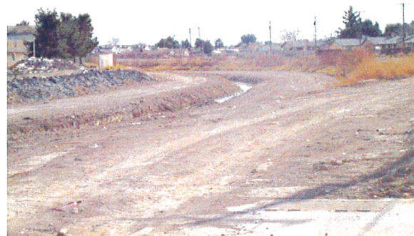
Las Vegas Wash south of Owens Avenue looking south.
