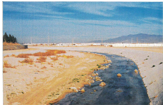
Las Vegas Wash at Vegas Valley Drive on top of bridge looking north. Note sedimentation along west bank.
