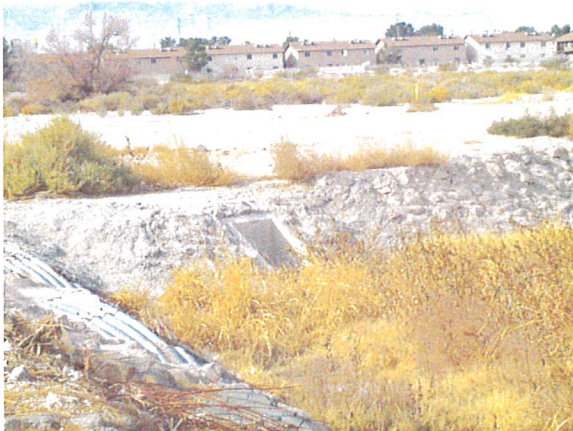
Las Vegas Wash at Cheyenne Avenue looking west at outlet structure on north side of road.
