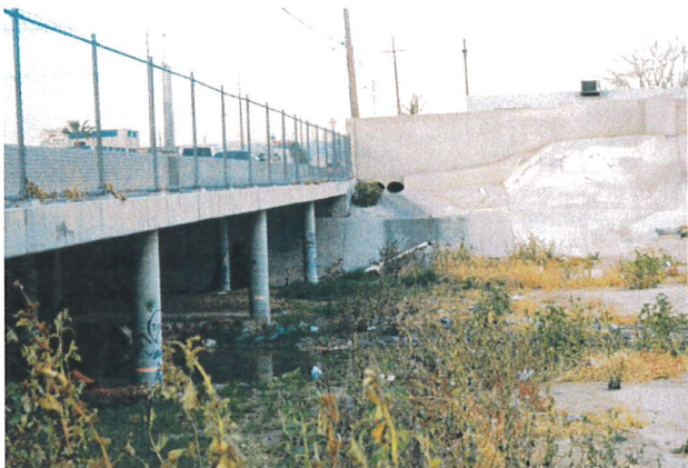
Las Vegas Wash north of Charleston Boulevard bridge looking west at storm drain outfall.
