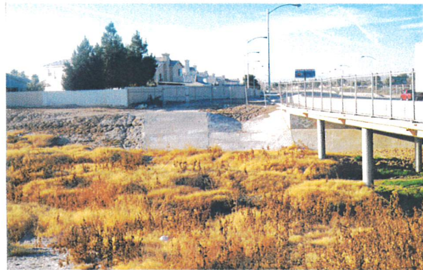
Las Vegas Wash at Nellis Boulevard looking south at channel access and east bridge face.
