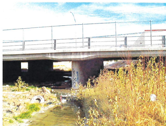
Las Vegas Wash looking east at west bridge face of Lamb Boulevard.
