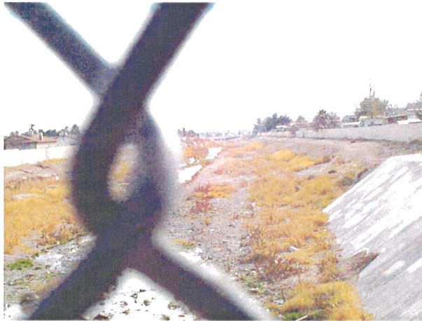
Las Vegas Wash at Carey Avenue looking south through chain-link fence.
