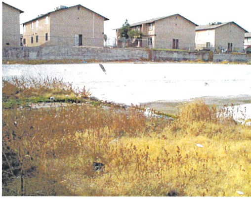
Las Vegas Wash at Civic Center Drive looking west at channel lining on northwest side of bridge. Note end of concrete lining.
