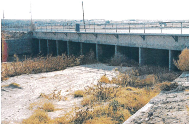
Las Vegas Wash at Vegas Valley Drive looking southeast at north culvert face.
