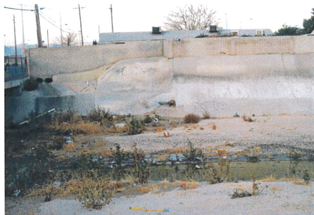
Las Vegas Wash north of Charleston Boulevard bridge looking west at sanitary sewer manhole.
