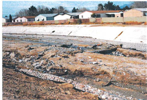
Las Vegas Wash north of Washington Avenue looking northwest. Note installation of gabions on south bank, cable-concrete block over sanitary sewer, drop structure and concrete lining on north bank.
