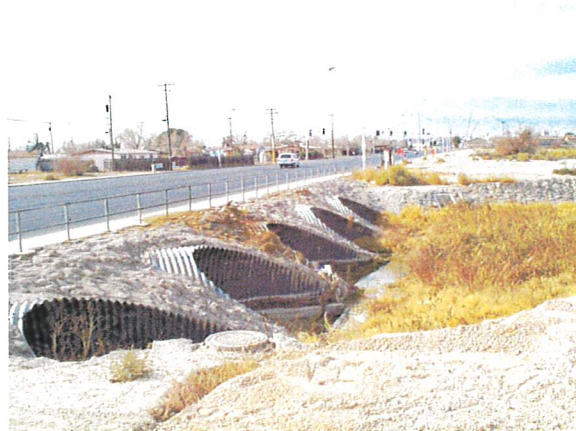
Las Vegas Wash at Cheyenne Avenue looking west at north culvert face.
