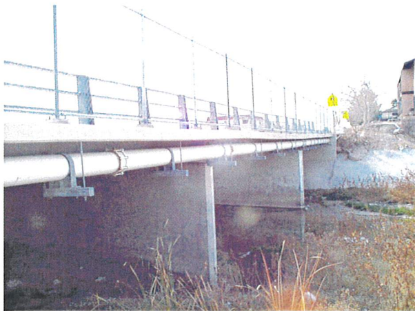
Las Vegas Wash at Civic Center Drive looking southwest at northwest bridge face.
