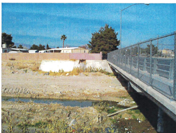
Las Vegas Wash at Lamb Boulevard looking north at west bridge face.
