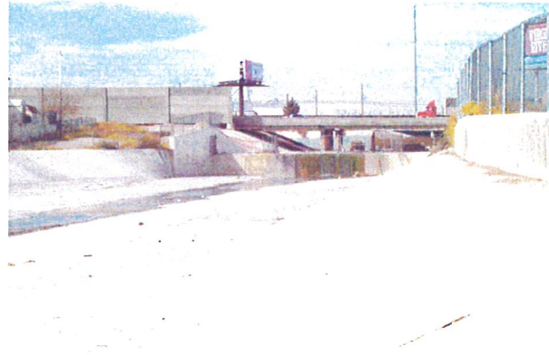
Las Vegas Wash at Civic Center Drive looking northwest towards I-15. Note drop structure.
