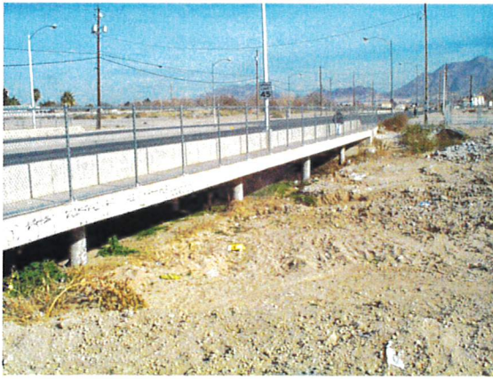
Las Vegas Wash looking northeast at south face of Owens Avenue bridge.
