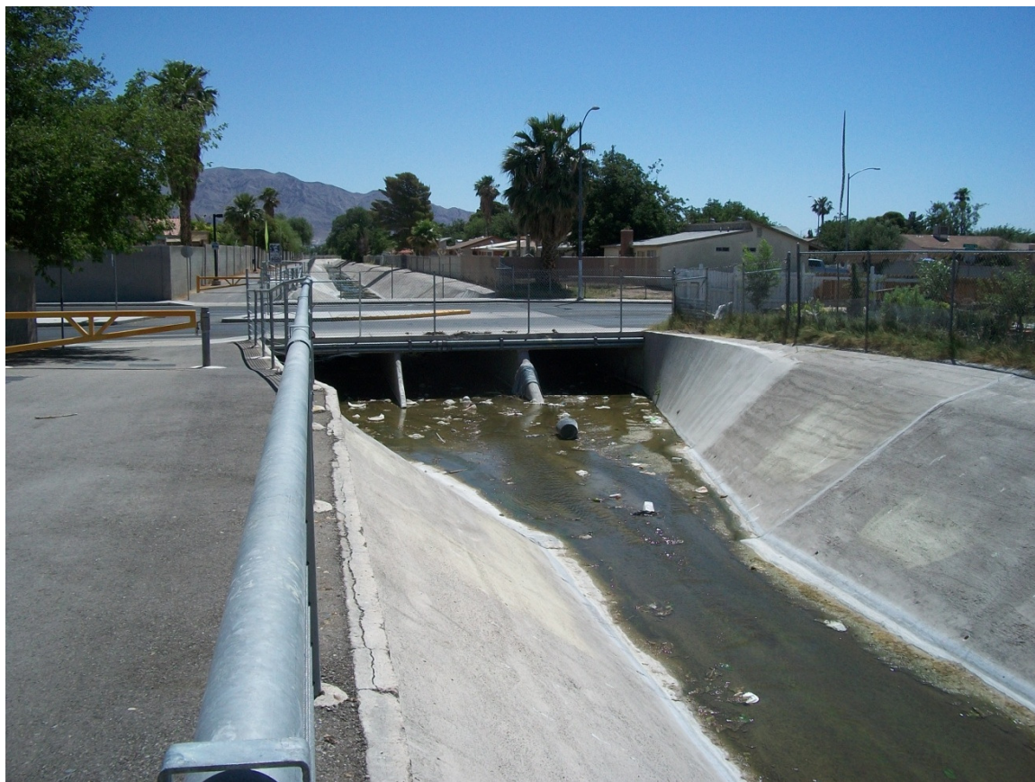
Photo 7: Looking east at the Cedar channel upstream of Sandhill Road crossing
