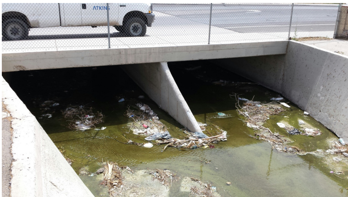
Photo 14: Looking east at the upstream face of Marion Street crossing
