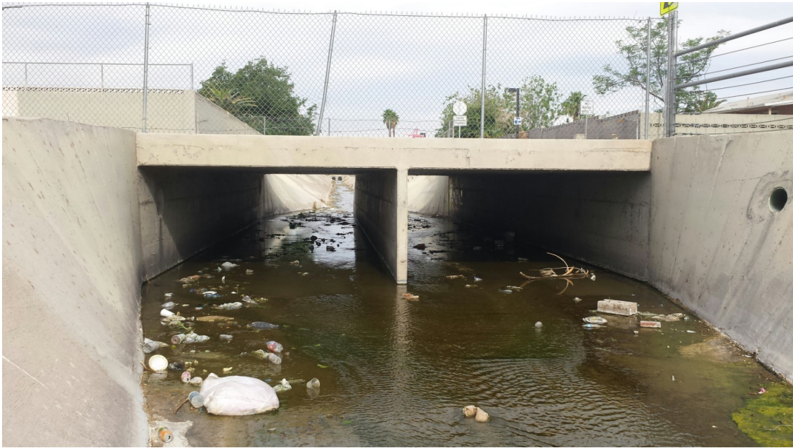
Photo 5: Looking west at the downstream face of Honolulu Street crossing
