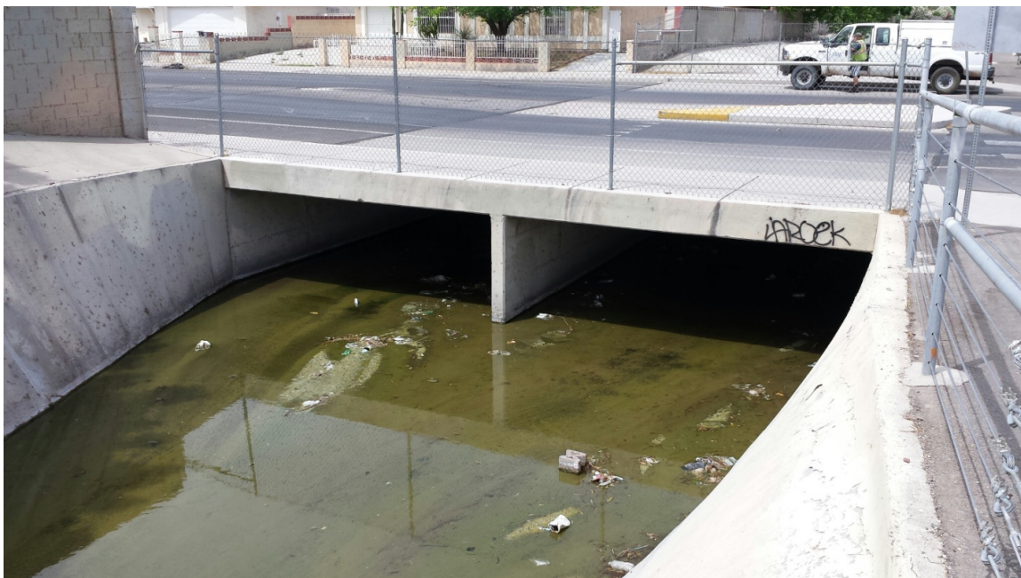
Photo 15: Looking west at the downstream face of Marion Street crossing
