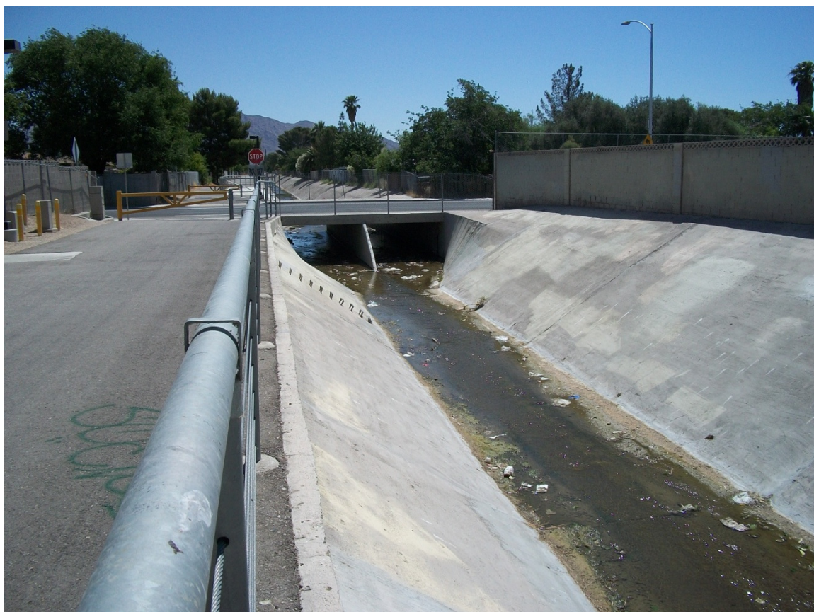
Photo 3: Looking east at the Cedar channel upstream of Honolulu Street crossing
