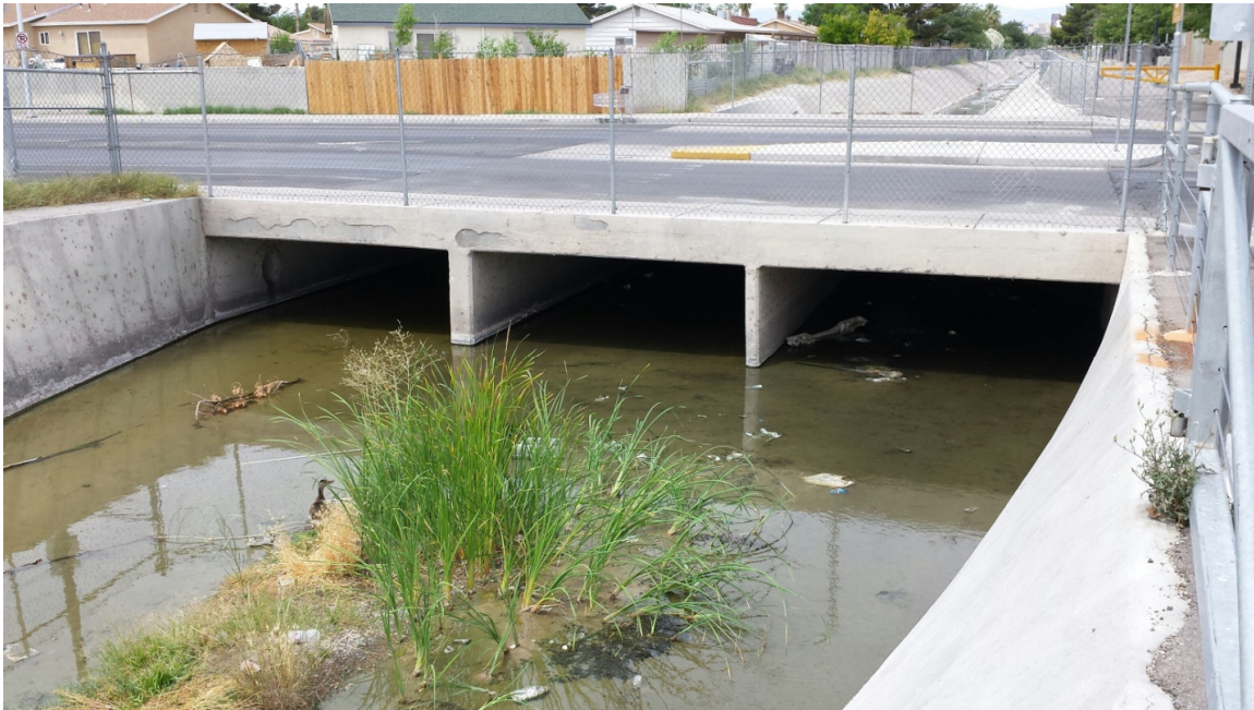
Photo 9: Looking west at the downstream face of Sandhill Road crossing
