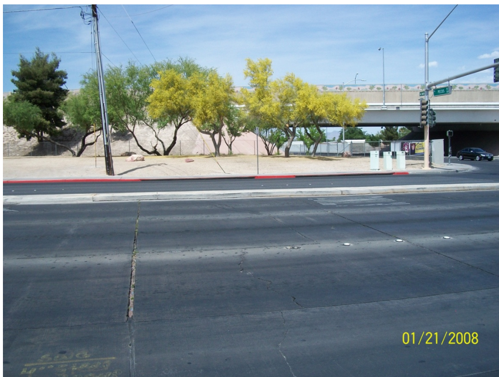
Photo 18: Looking north at drop inlets on Stewart Ave, west of Pecos Rd
