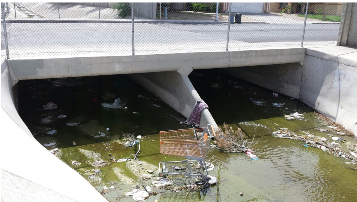
Photo 16: Looking east at the upstream face of Page Street crossing
