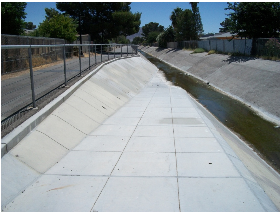
Photo 20: Looking east at channel access ramp east of Honolulu St
