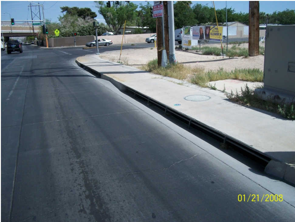
Photo 19: Looking east at drop inlets on south side of Stewart Ave, west of Pecos Rd
