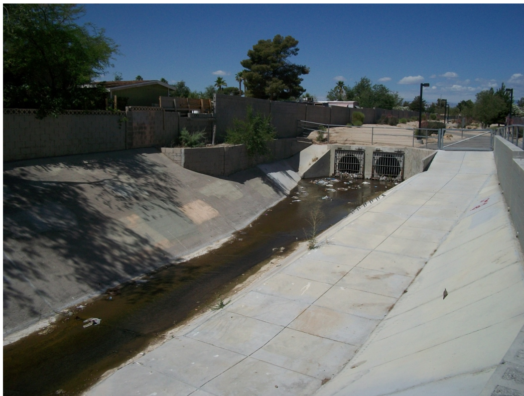
Photo 1: Looking at the upstream end of the channel at the two (2) 72-inch RCP's
