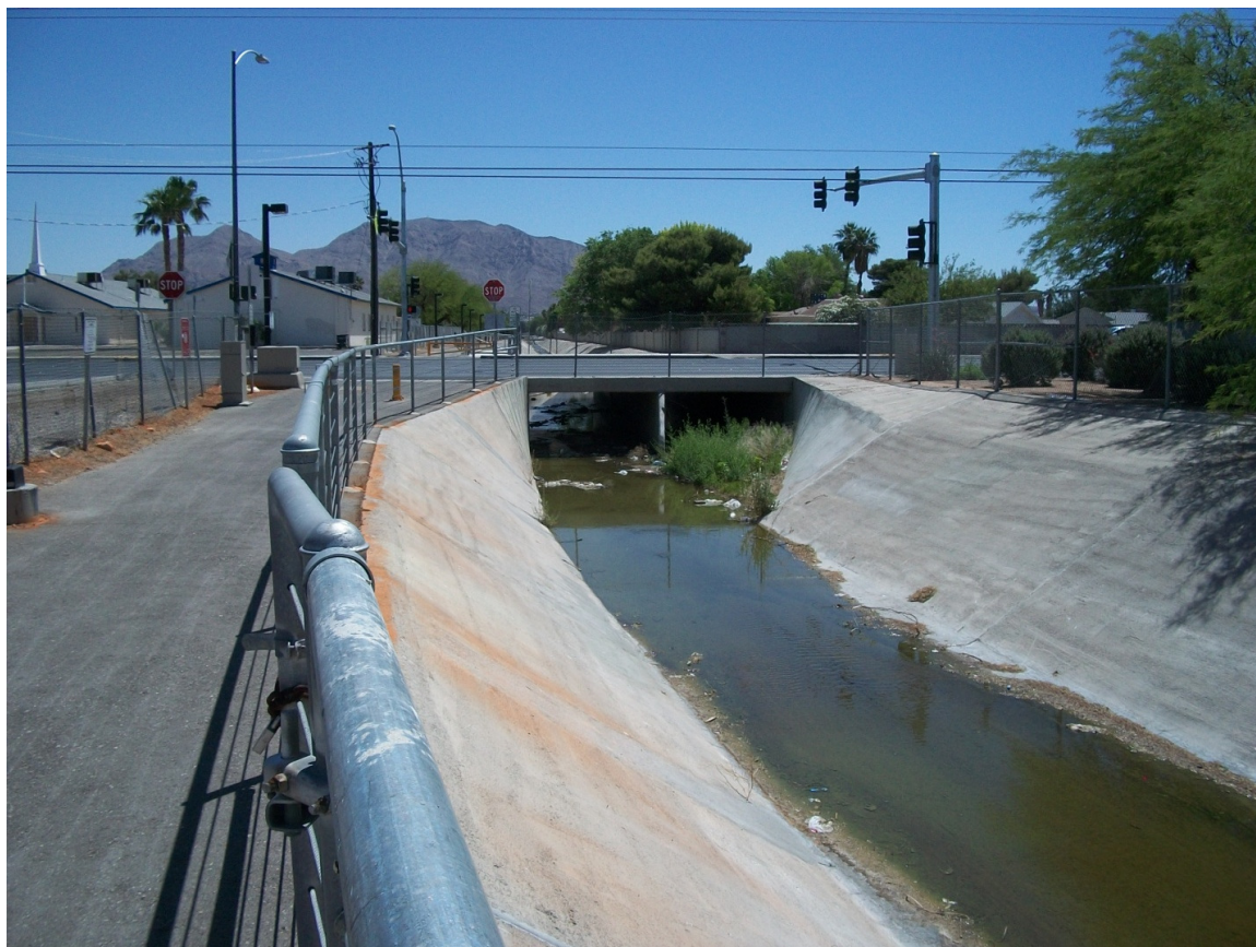
Photo 11: Looking east at the Cedar channel upstream of Lamb Boulevard crossing
