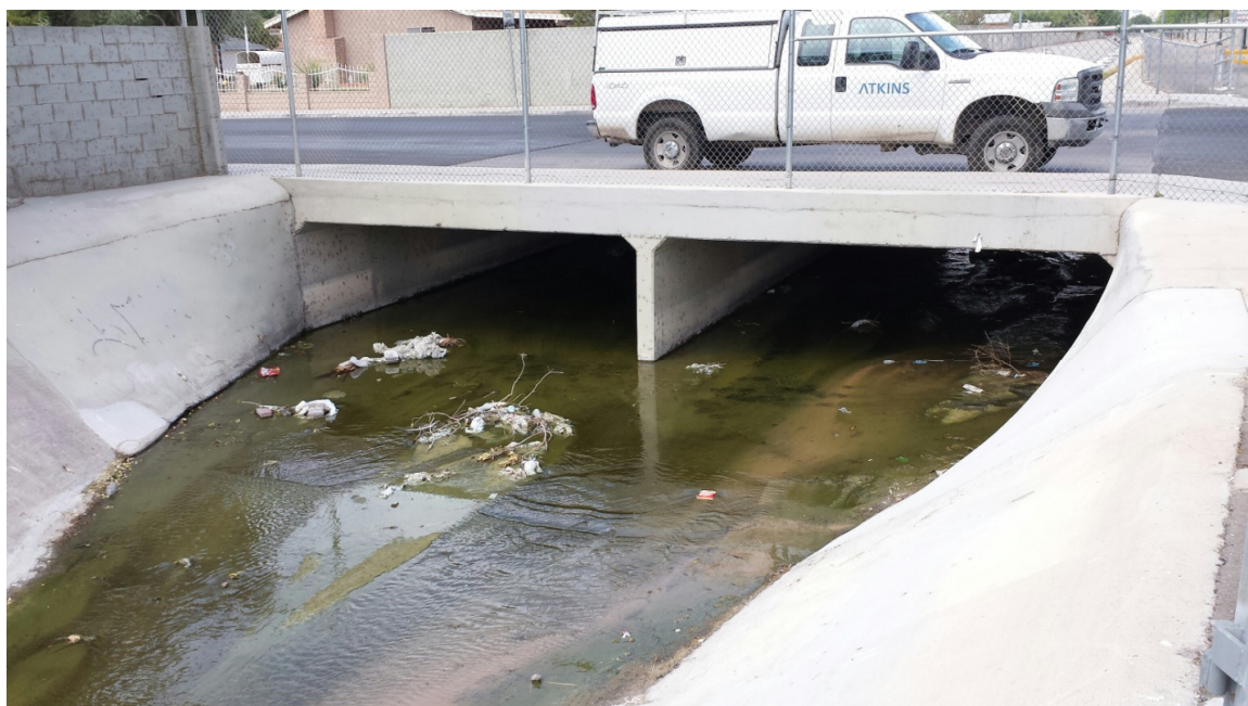
Photo 17: Looking west at the downstream face of Page Street crossing
