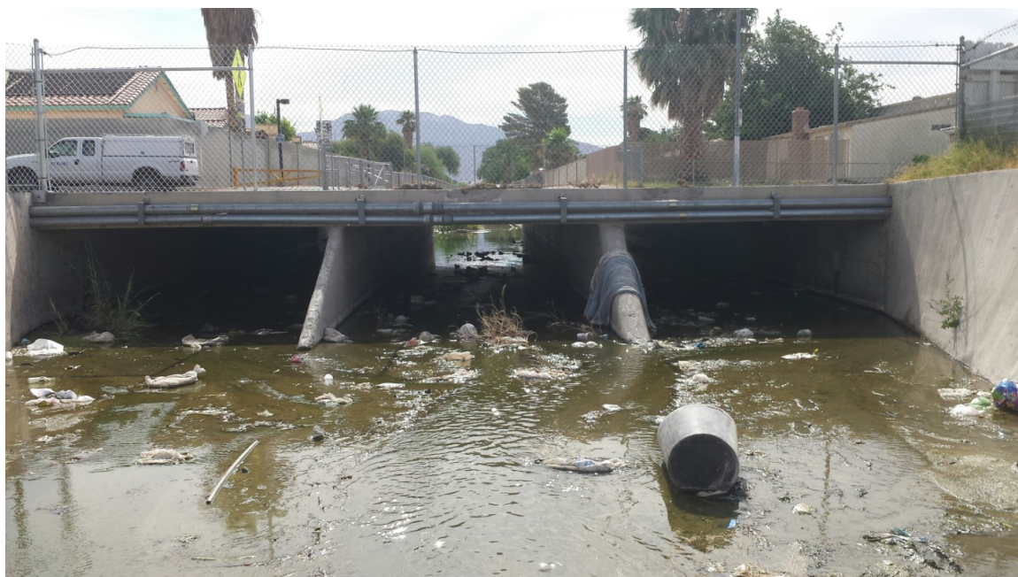
Photo 8: Looking east at the upstream face of Sandhill Road crossing
