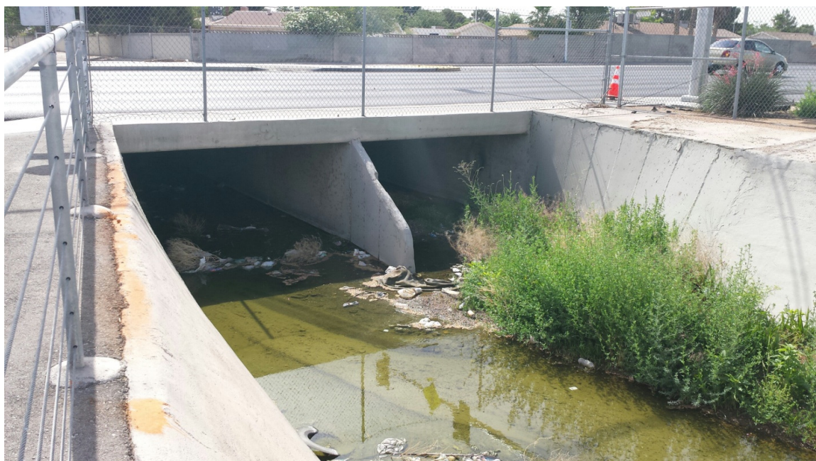
Photo 12: Looking east at the upstream face of Lamb Boulevard crossing
