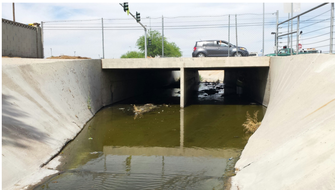
Photo 13: Looking west at the downstream face of Lamb Boulevard crossing
