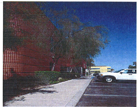
Viewpoint H away from building looking North
