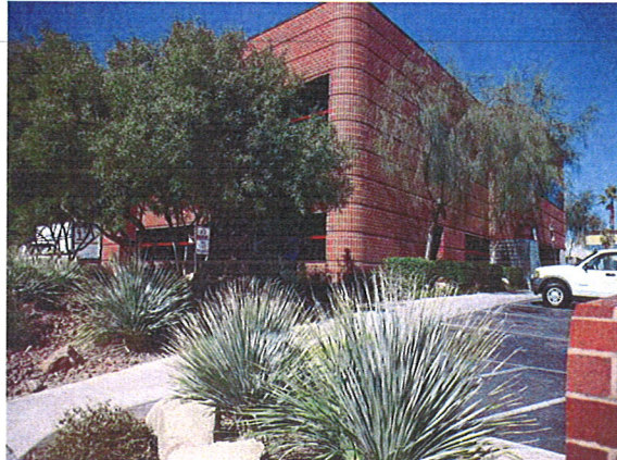
Viewpoint E looking Northwest
