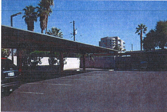
Viewpoint A looking Northeast
