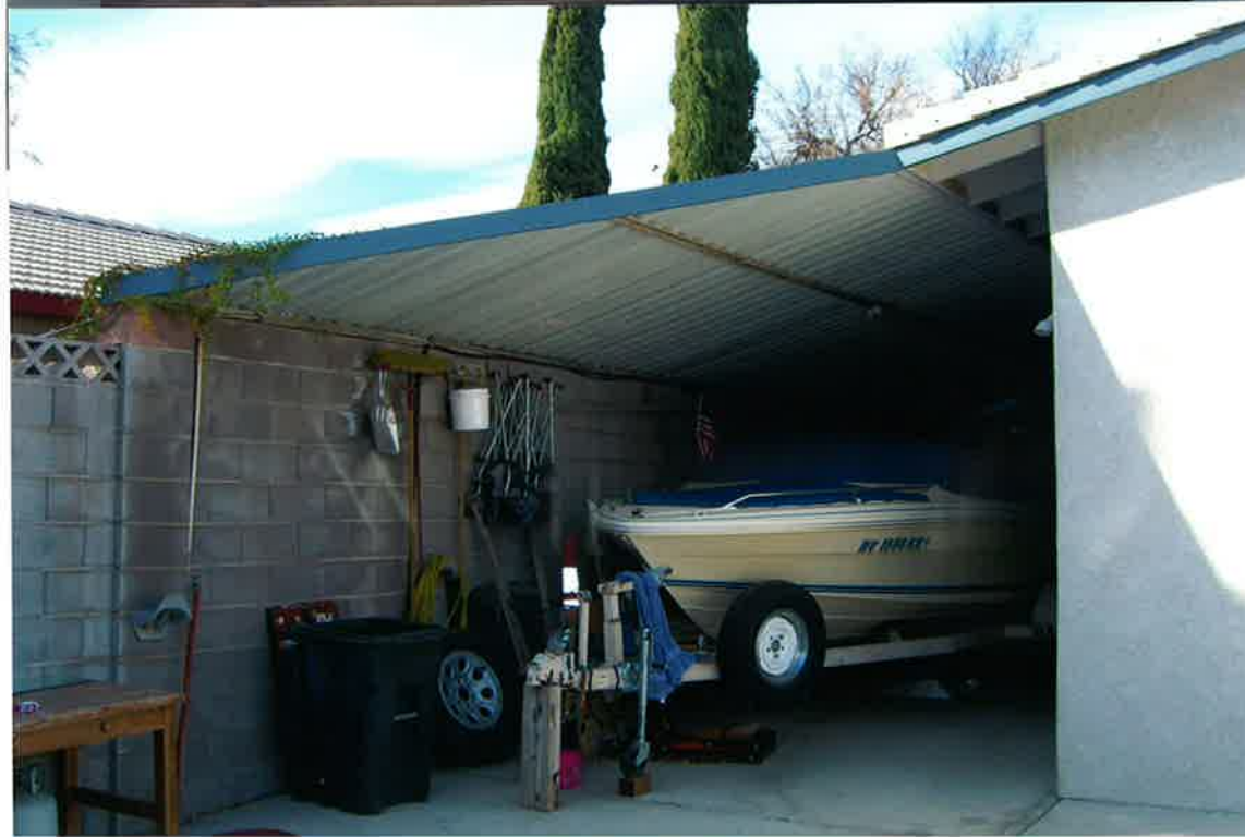
Awning South Side Rear
