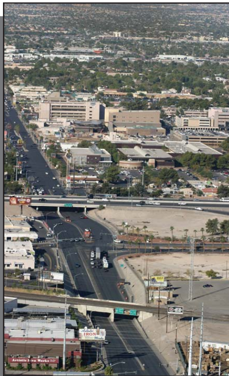
Charleston Boulevard looking west towards I-15.
