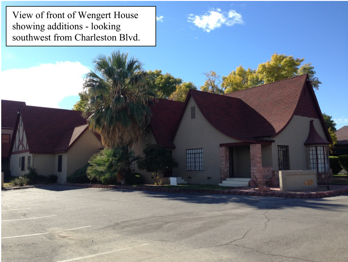
View of front of Wengert House showing additions - looking southwest from Charleston Blvd.
