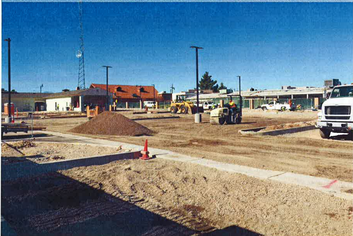
Preparing lot for new pavement
