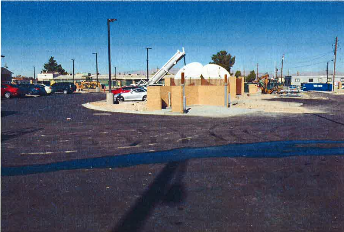
Re-paved parking lot and new location for satellite equipment
