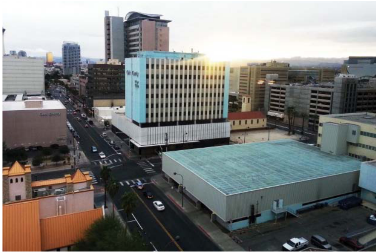
The Bridger Building
