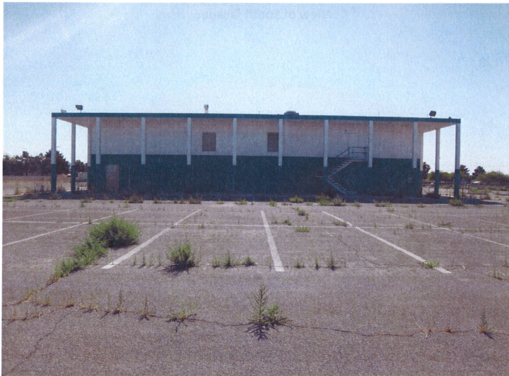
View of West façade.
