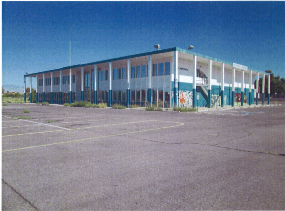
View looking NW of SW corner of the building.
