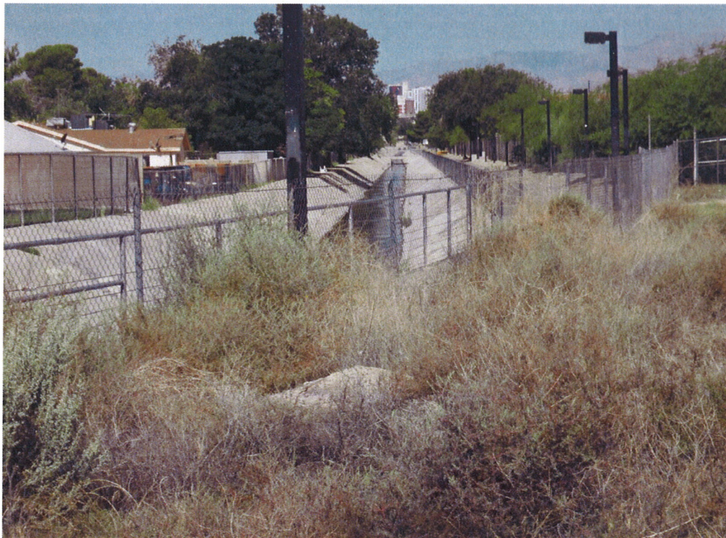
K. View of drainage ditch and multi-use pathway that runs along the South side of the property.
