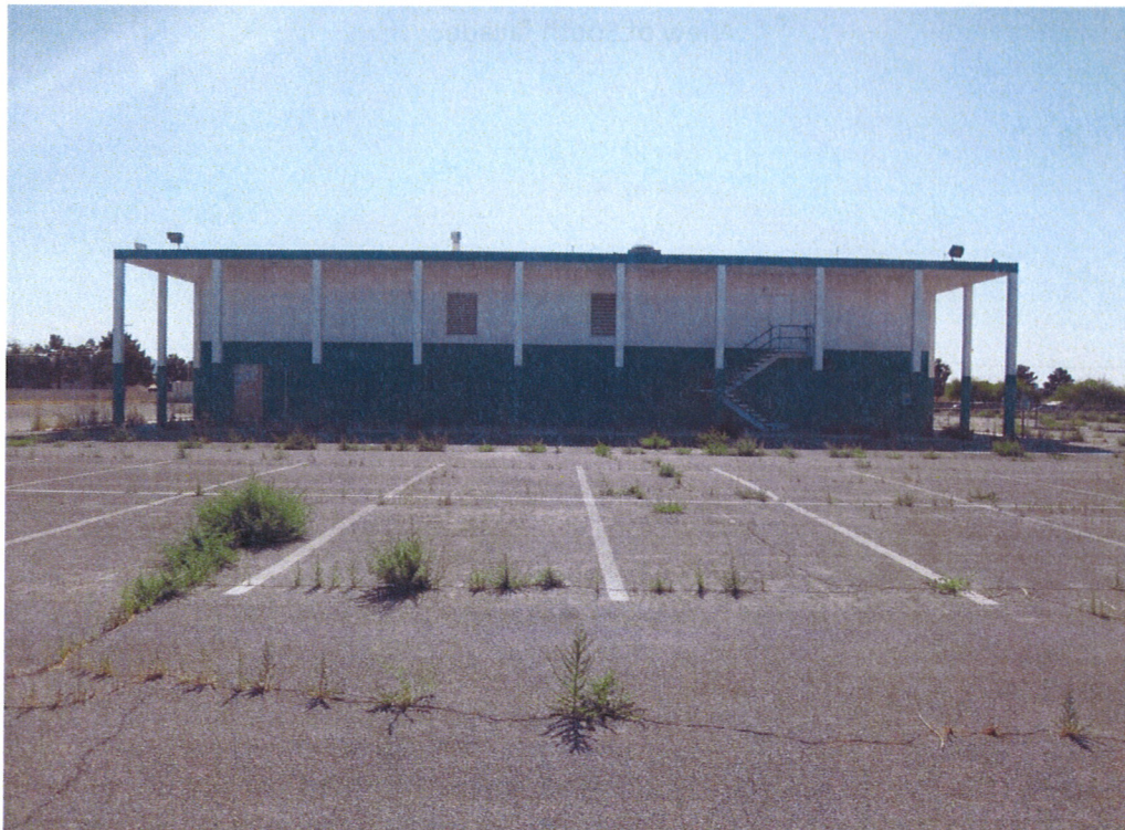
View of West façade.
