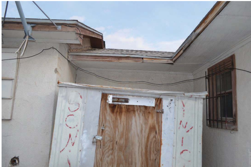
Harrison's Guest House, connector between guest house and northernmost addition, facing north. 19 December 2013
