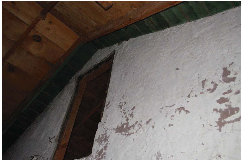
Harrison's Guest House, original stucco on rear façade, visible from the rear porch. 19 December 2013
