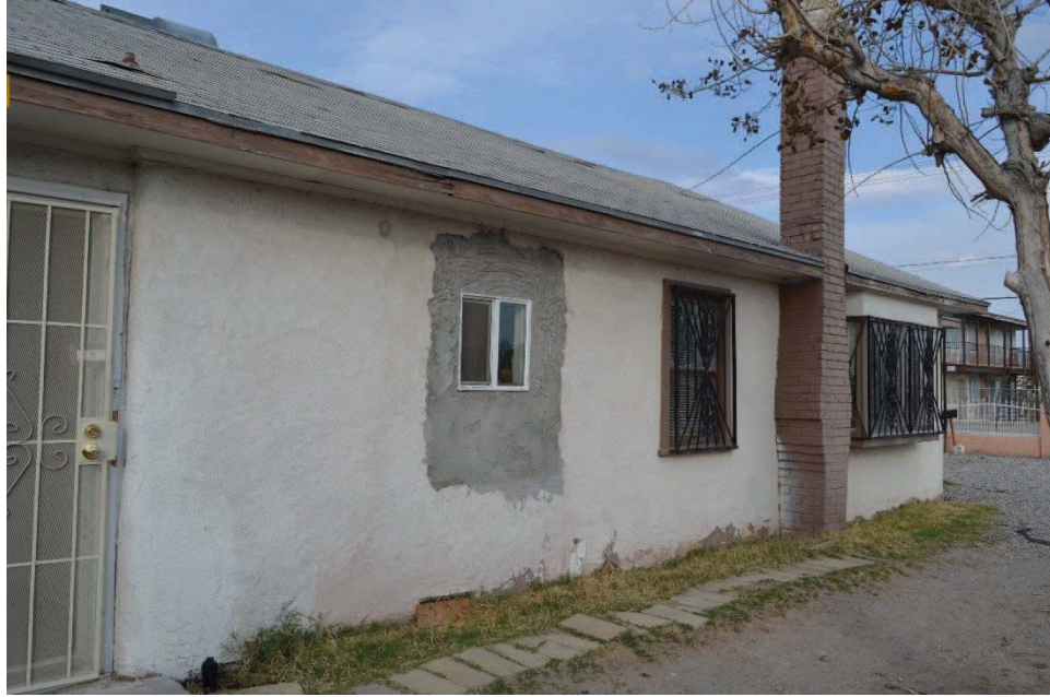
Harrison's Guest House, south elevation of original bungalow showing modern modifications, facing northeast. 19 December 2013
