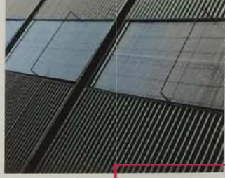
Corrugated Metal Panels
