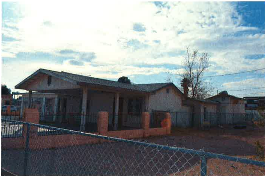
Harrison's Guest House, north elevation showing additions, facing southwest. The guest house is in the rear view. 19 December 2013
