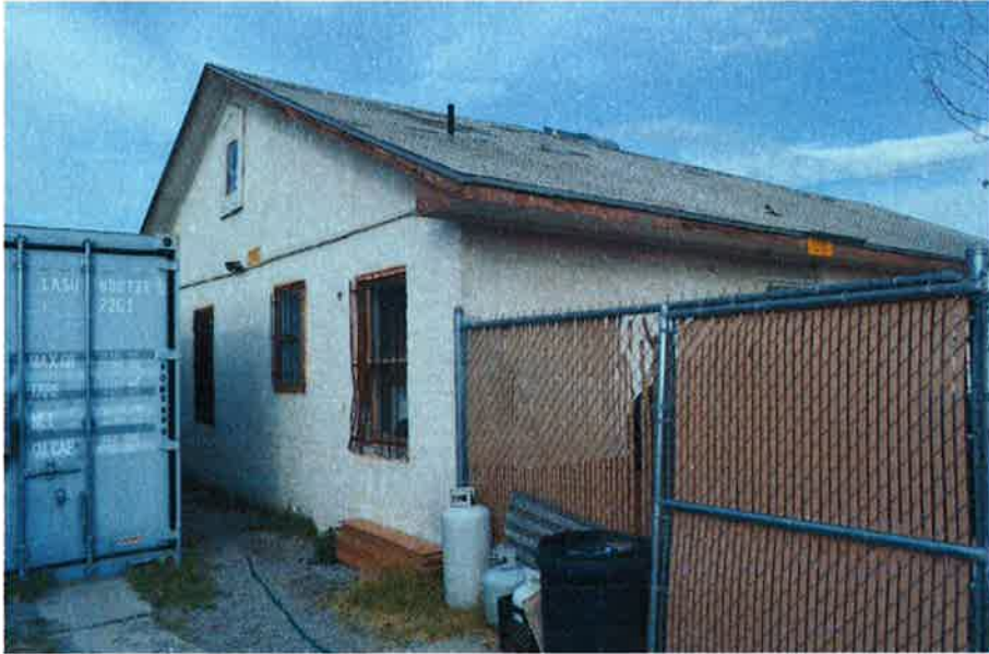
Harrison's Guest House, west (rear) elevation showing the first of the additions, facing northeast. 19 December 2013
