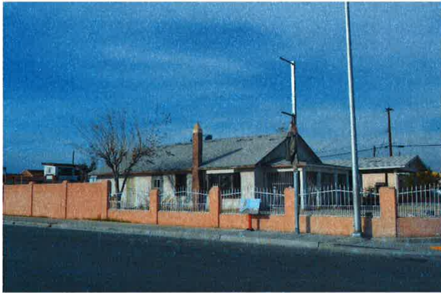
Harrison's Guest House, south elevation, facing northwest. Original bungalow in front view. 19 December 2013
