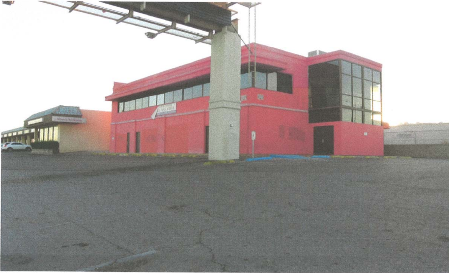
Main view of the building complex facing south from the driveway on neighbors side.
