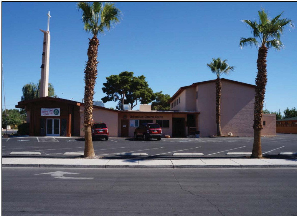
Photograph 49. Reformation Lutheran Church, showing the large two-story addition at the southern end of the building, facing east.
