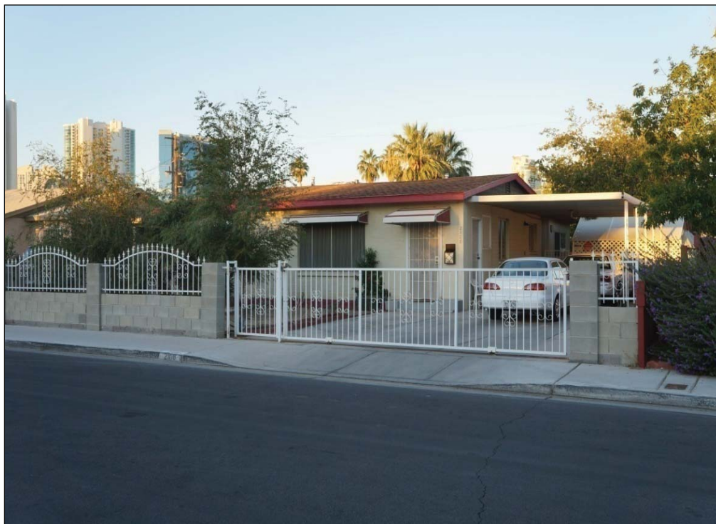
Photograph 20. Example of a "Plan A" style home at 2108 Beverly Way, facing southwest.
