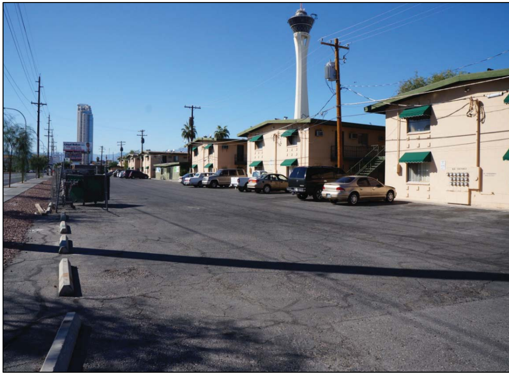
Photograph 3. East Park Apartments, a 96-unit apartment complex at 500–520 San Pablo Drive, facing northwest.
