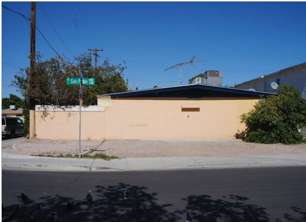
Photograph 35. 2303–2309 Santa Rosa Drive, a multi-family dwelling or four-plex built in the Post-WWII/Ranch architectural style, facing north.
