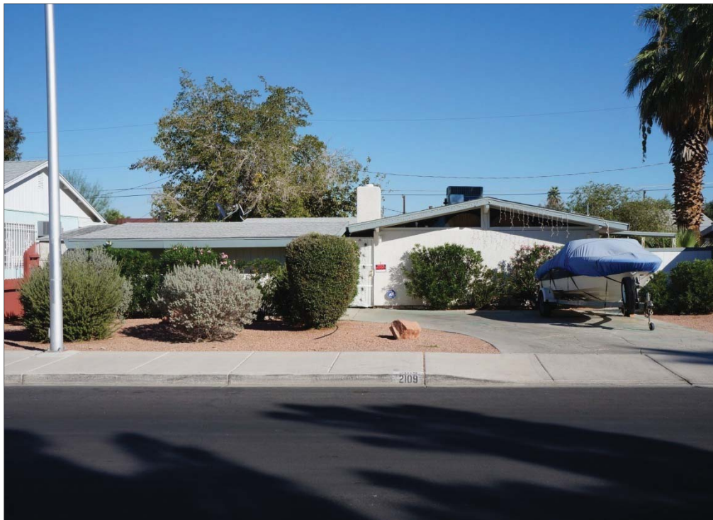
Photograph 25. Wood frame and stucco single family dwelling at 2109 Van Patten Place, constructed in the Post-WWII/Contemporary style, facing east.
