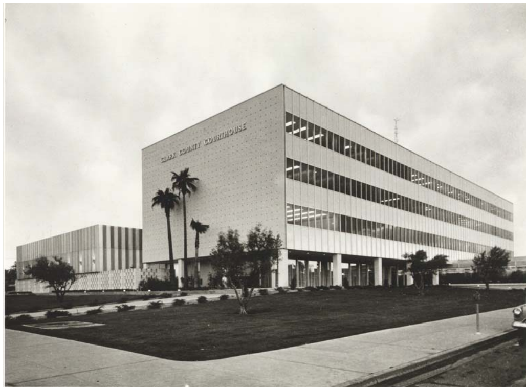
Photograph 7. Clark County Courthouse designed by Zick and Sharp in 1958 (Image courtesy of UNLV Libraries).
