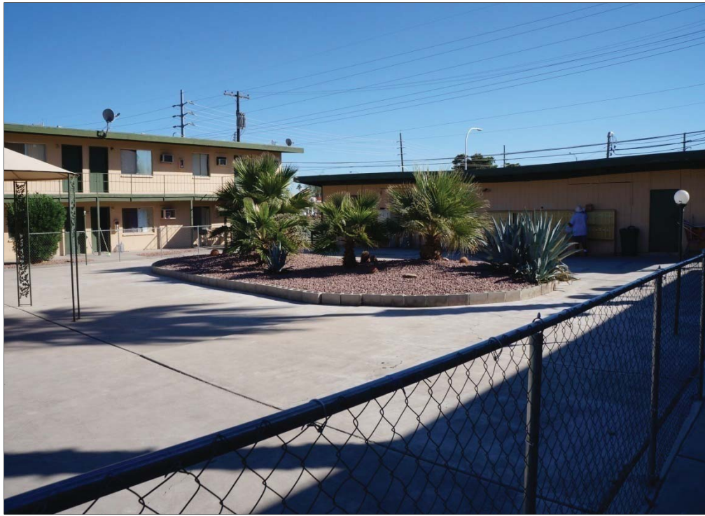
Photograph 42. Storage building located at the center of the Park East Apartment, facing southeast. Note the landscaped “island” in the center of the courtyard which was originally a swimming pool.
