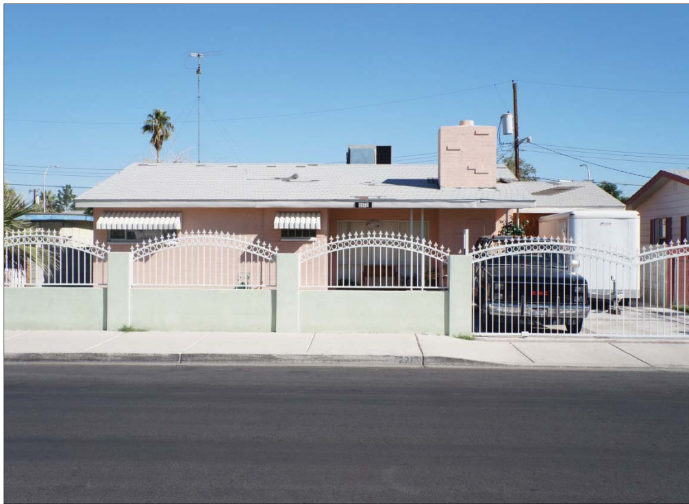
Photograph 30. Example of single family dwelling at 2217 Van Patten Place designed in the Post-WWII/Ranch architectural style, facing east.
