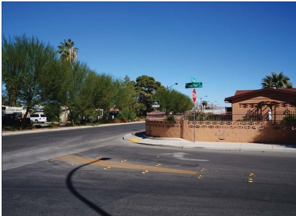
Photograph 51. Example of a raised sidewalk ramp at the southeast corner of East Saint Louis Avenue and Santa Ynez Drive, facing southeast.
