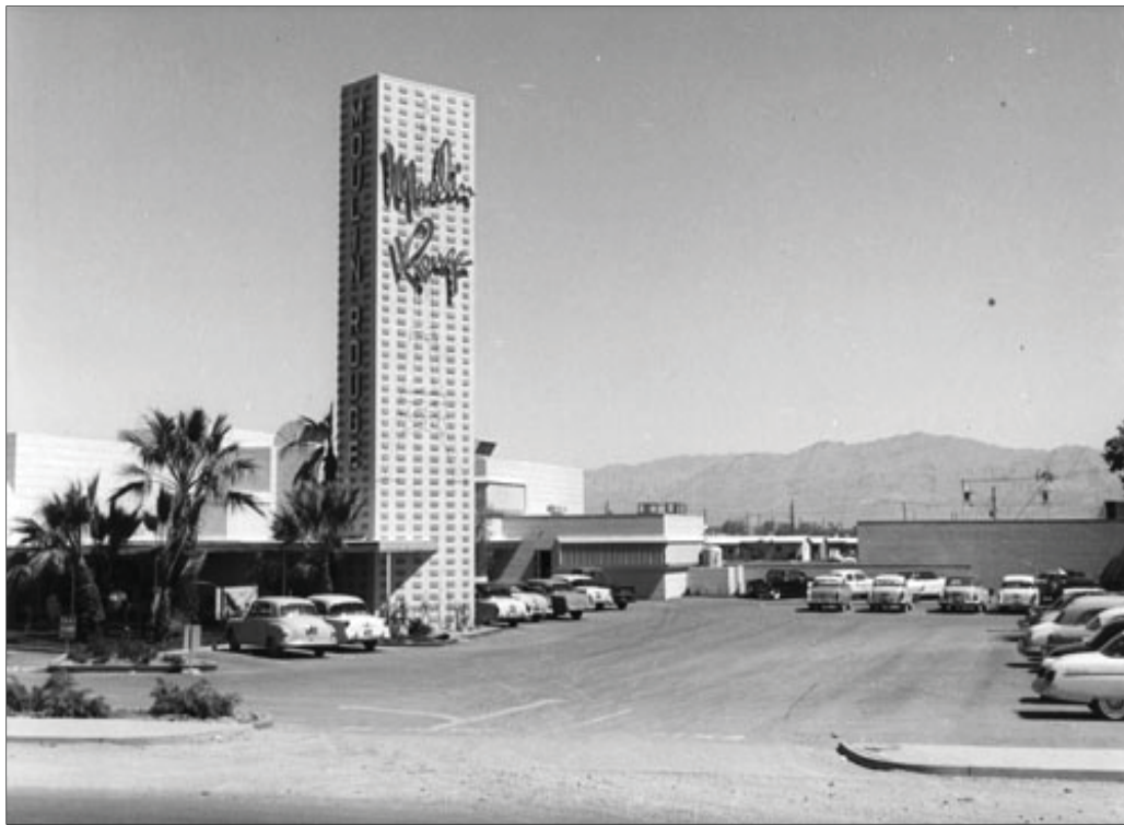
Photograph 5. The Moulin Rouge Hotel designed by Zick and Sharp in 1955 (Image courtesy of UNLV Special Collections).
