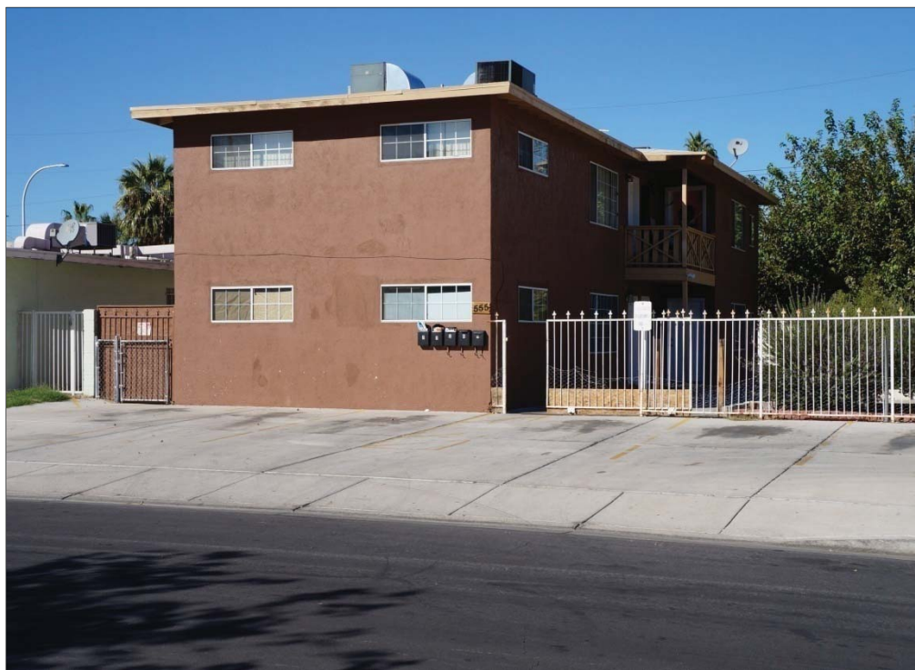
Photograph 23. Wood frame and stucco four-plex at 555 San Pablo Drive, facing northwest.
