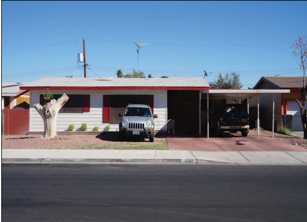
Photograph 22. Example of a "Plan C" style home at 2301 Van Patten Place, facing east.
