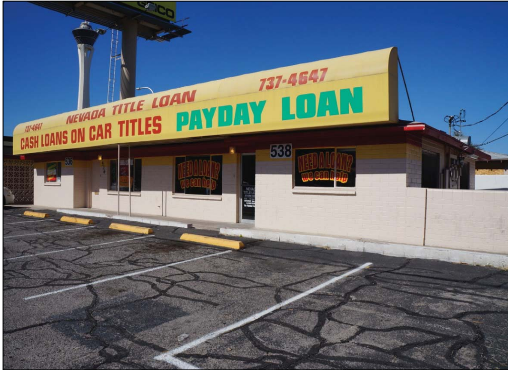
Photograph 47. 536-538 East Sahara Avenue, duplex converted to a commercial property, looking northwest.
