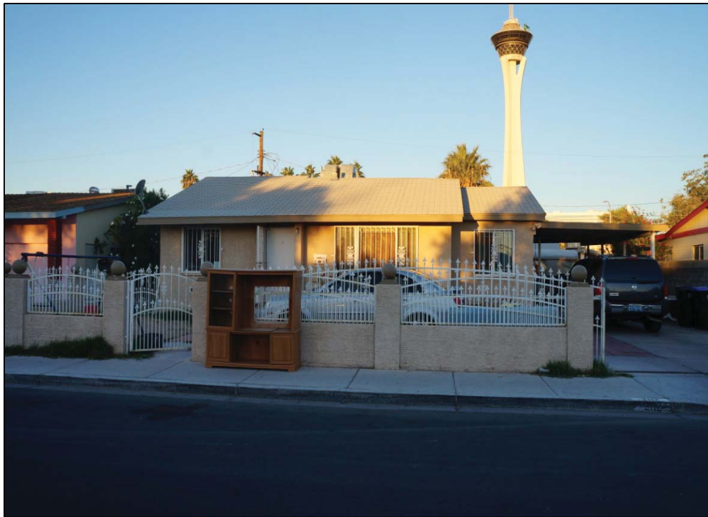
Photograph 59. 2112 Beverly Way, an example of an ineligible building with stucco sheathing and vinyl windows, facing west.
