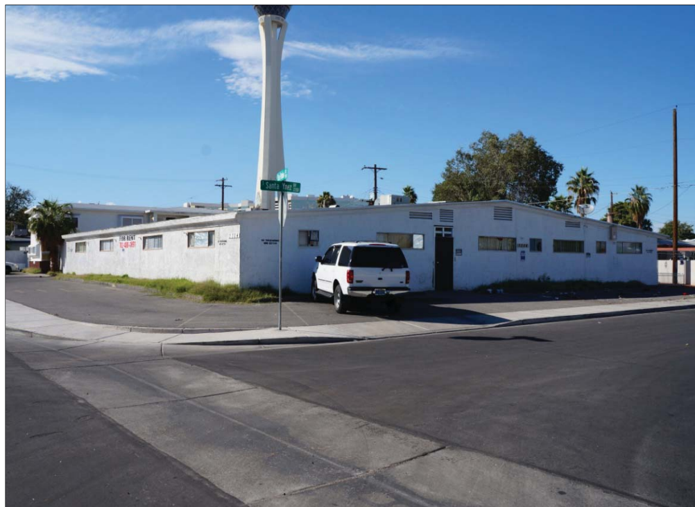
Photograph 19. 2304 Santa Ynez Drive, designed by Moffitt and Hendricks in 1959, facing northwest.
