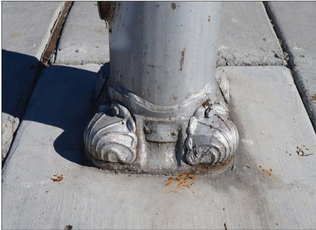
Photograph 57. Photograph showing decorative scroll detailing on the base of a historic street light on the south side of Santa Rosa Drive.
