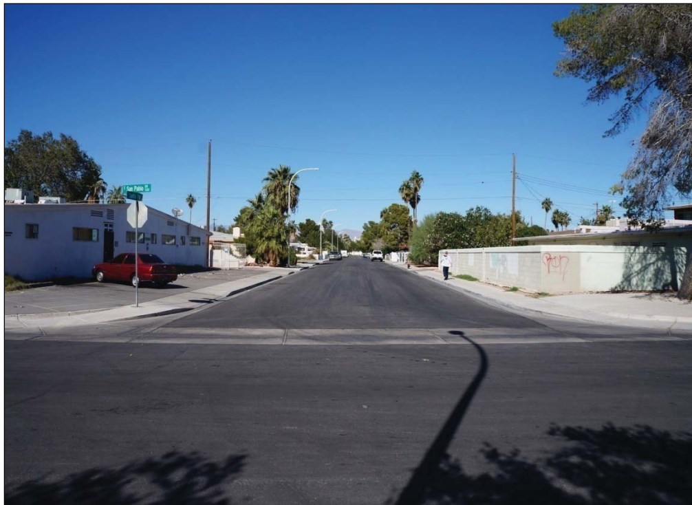
Photograph 56. Photograph showing a row of standard street lights along the west side of Santa Ynez Drive, facing north.
