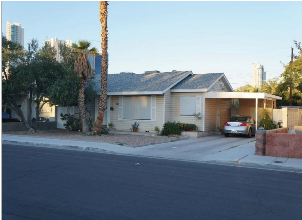
Photograph 44. Example of residence with a carport and rear concrete block storage building at 2212 Beverly Way, facing southwest.
