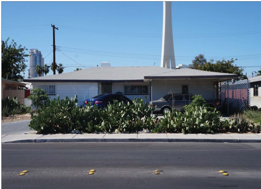
Photograph 45. Example of hipped roof carport projection at 2108 South Sixth Street, facing west.
