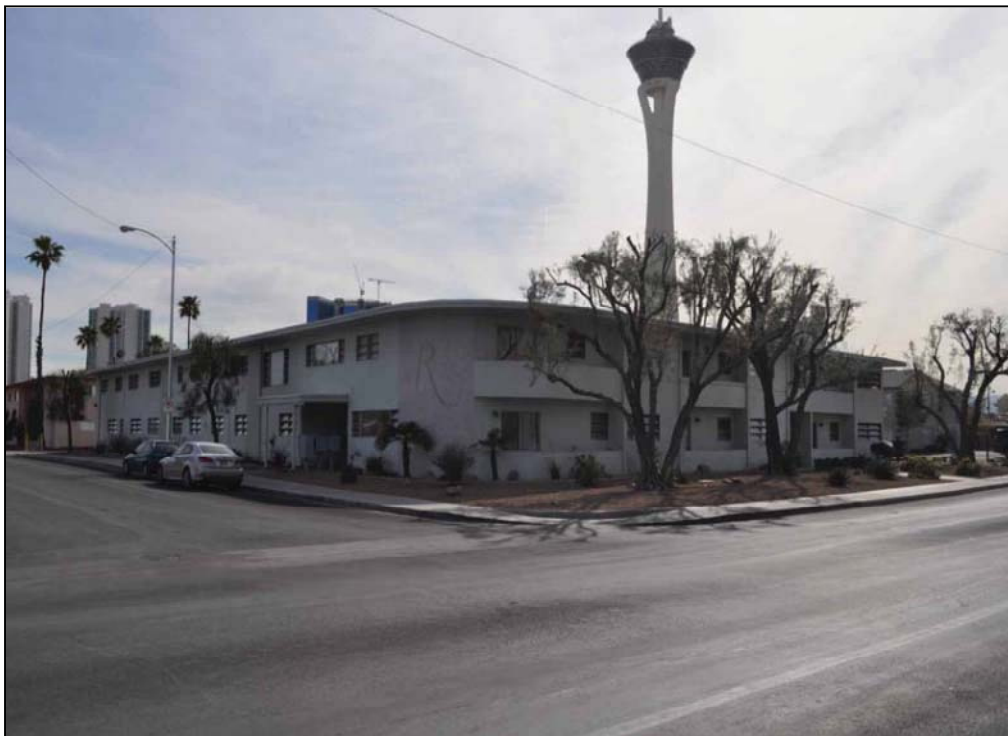
Photograph 2. The Rexford, a 92-unit apartment complex at 1700 Rexford Drive, located within the Phase I Beverly Green project area, facing southwest (Image reprinted from Harmon et al. 2011:41).
