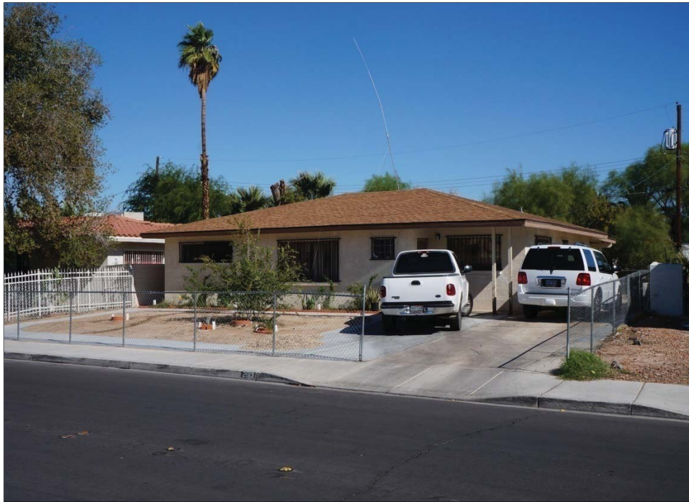
Photograph 55. Photograph showing a driveway at 2013 Santa Rosa Drive that has been widened to create off-street parking for multiple vehicles, facing northeast.
