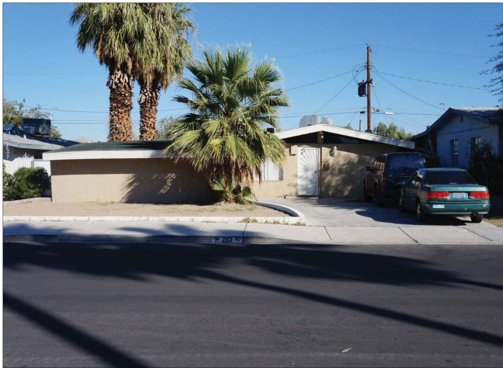
Photograph 24. Wood frame and stucco Post-WWII/Contemporary style home at 2113 Van Patten Place, facing east.
