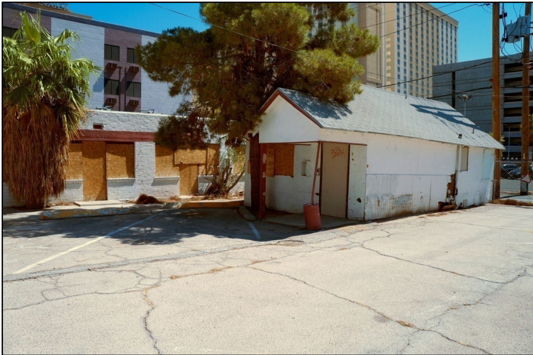
Photograph 4. Photograph showing the main (western) and southern facades of Building No. 3, constructed ca. 1928, facing southeast. Building No. 2 is visible in the background.
