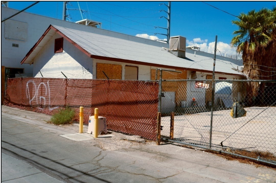
Photograph 5. Photograph showing the main (northern) and eastern facades of Building No. 4, constructed ca. 1928, facing southwest.
