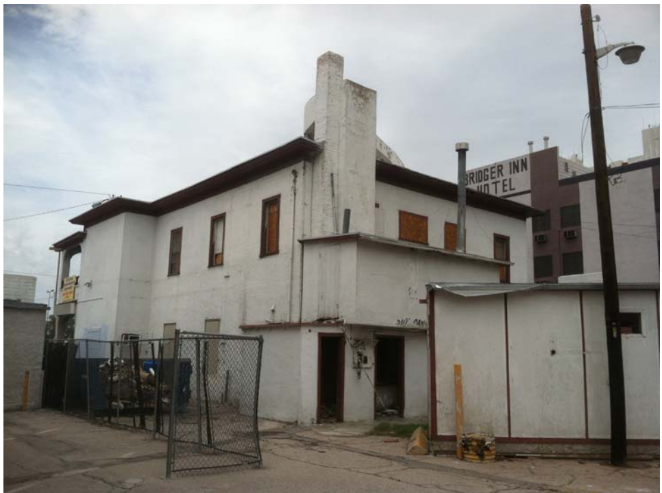
Photograph 4: View of south and west side of subject structure, facing northeast.
