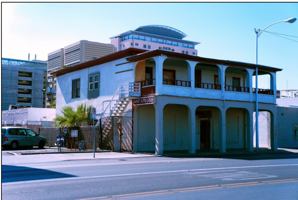
Photograph 1. Main (western) and northern facades of the Victory Hotel building, facing east.
