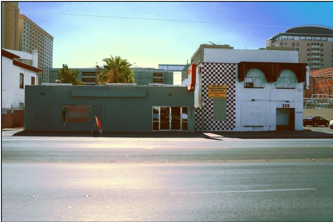
Photograph 6. Photograph showing the main (western) façade of Building No. 5 (at left), constructed ca. 1930, facing southeast. 319 S. Main Street, a two-story masonry building formally housing the Little Hotel rooming house is visible to the right of Building No. 5.
