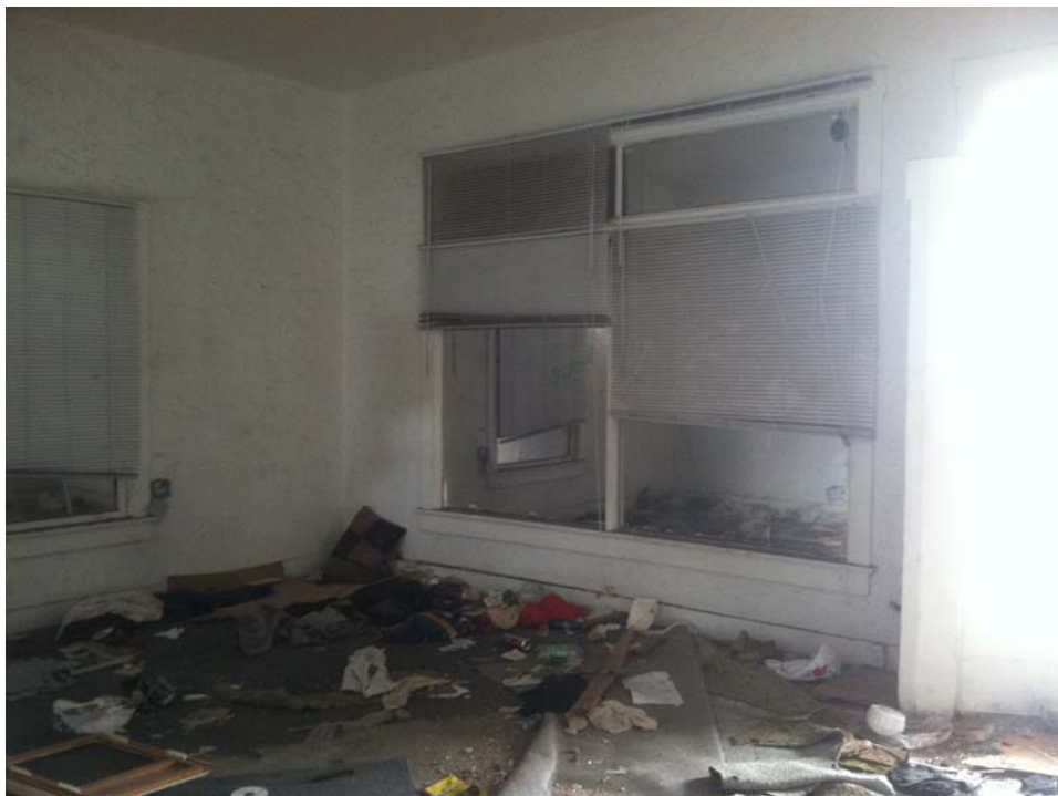
Photograph 5: View of lobby area of main structure.
