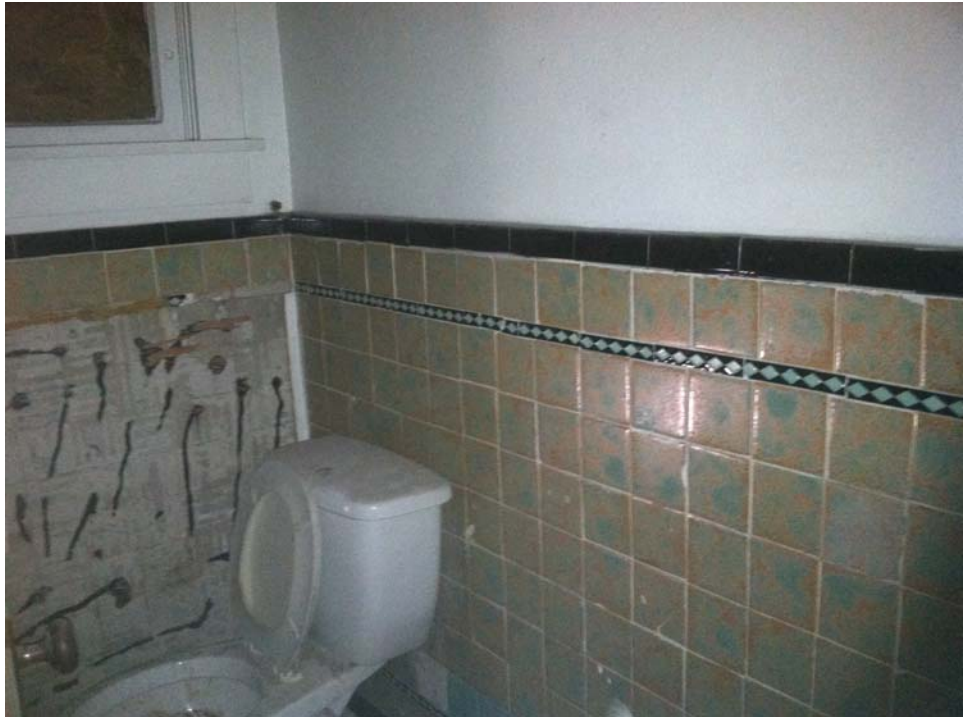
Photograph 7: View of the second floor common restroom wall with wall and bull nose tile.
