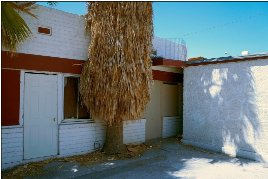
Photograph 7. Photograph showing the main (western) and southern facades of Building No. 6, constructed ca. 1930, facing southwest. An addition (possibly wood frame) to the rear of Building No. 5 is visible at right.
