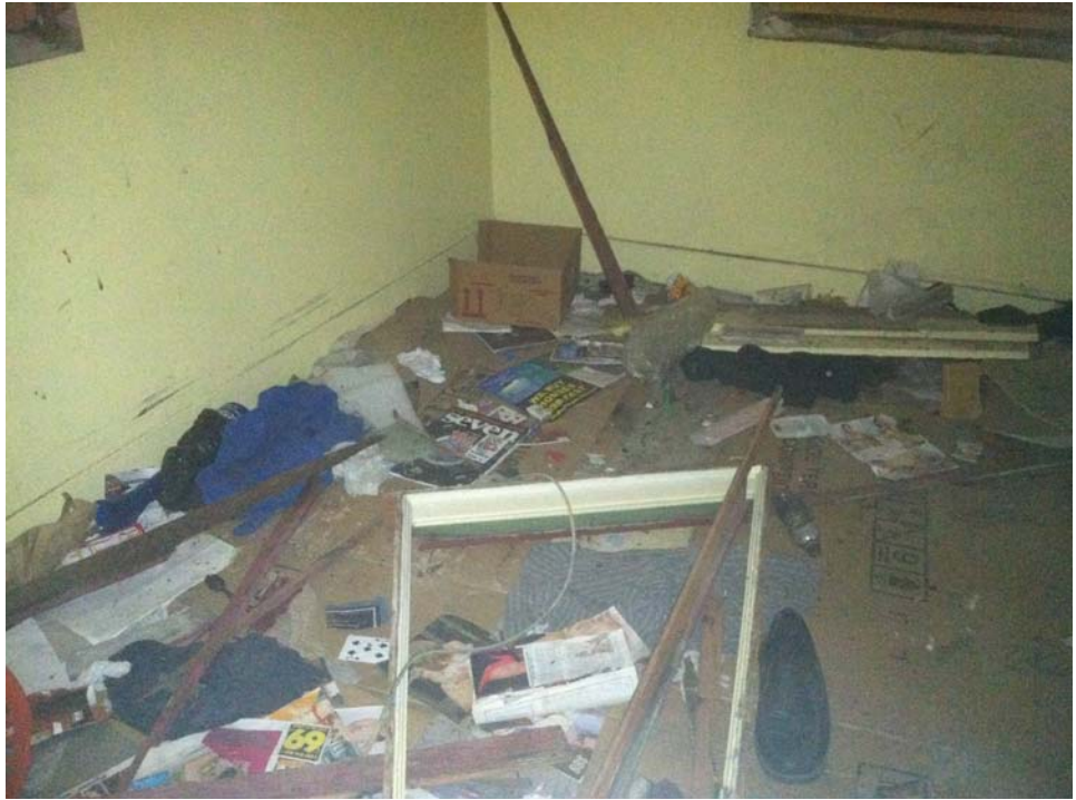
Photograph 9: View of window frame debris in Room 4.
