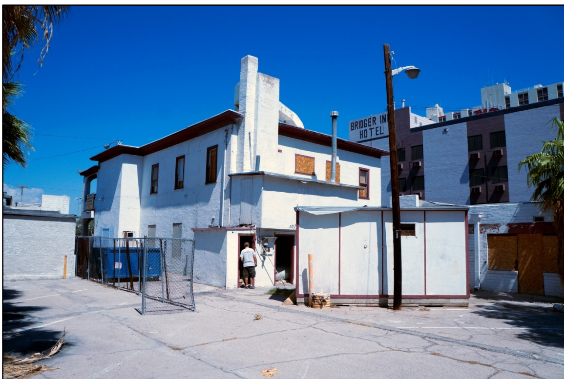
Photograph 2. Rear (eastern) and southern facades of the Victory Hotel building, facing northwest.
