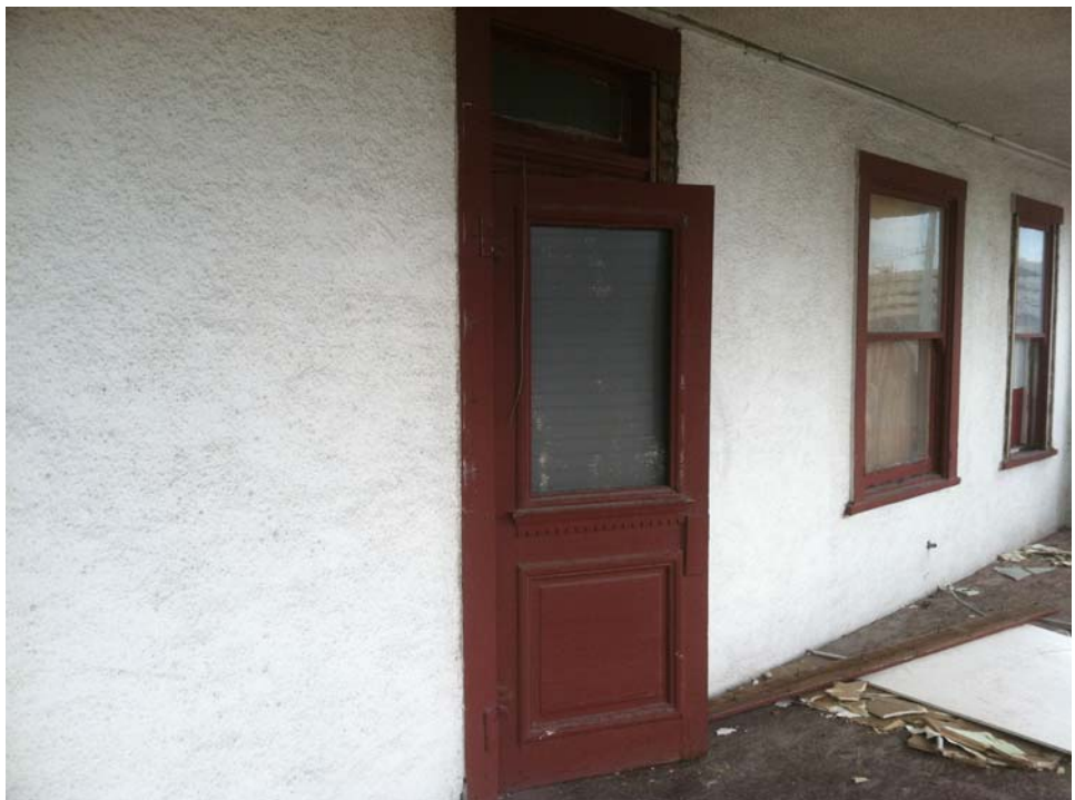
Photograph 10: View of exterior balcony door and south window.
