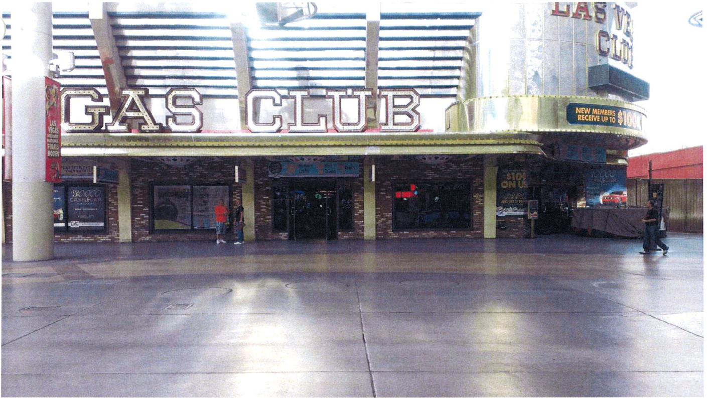
Before Pictures (ARELNI, LLC – 18 Fremont Street)
