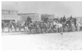
Freight Wagon on Fremont Street
