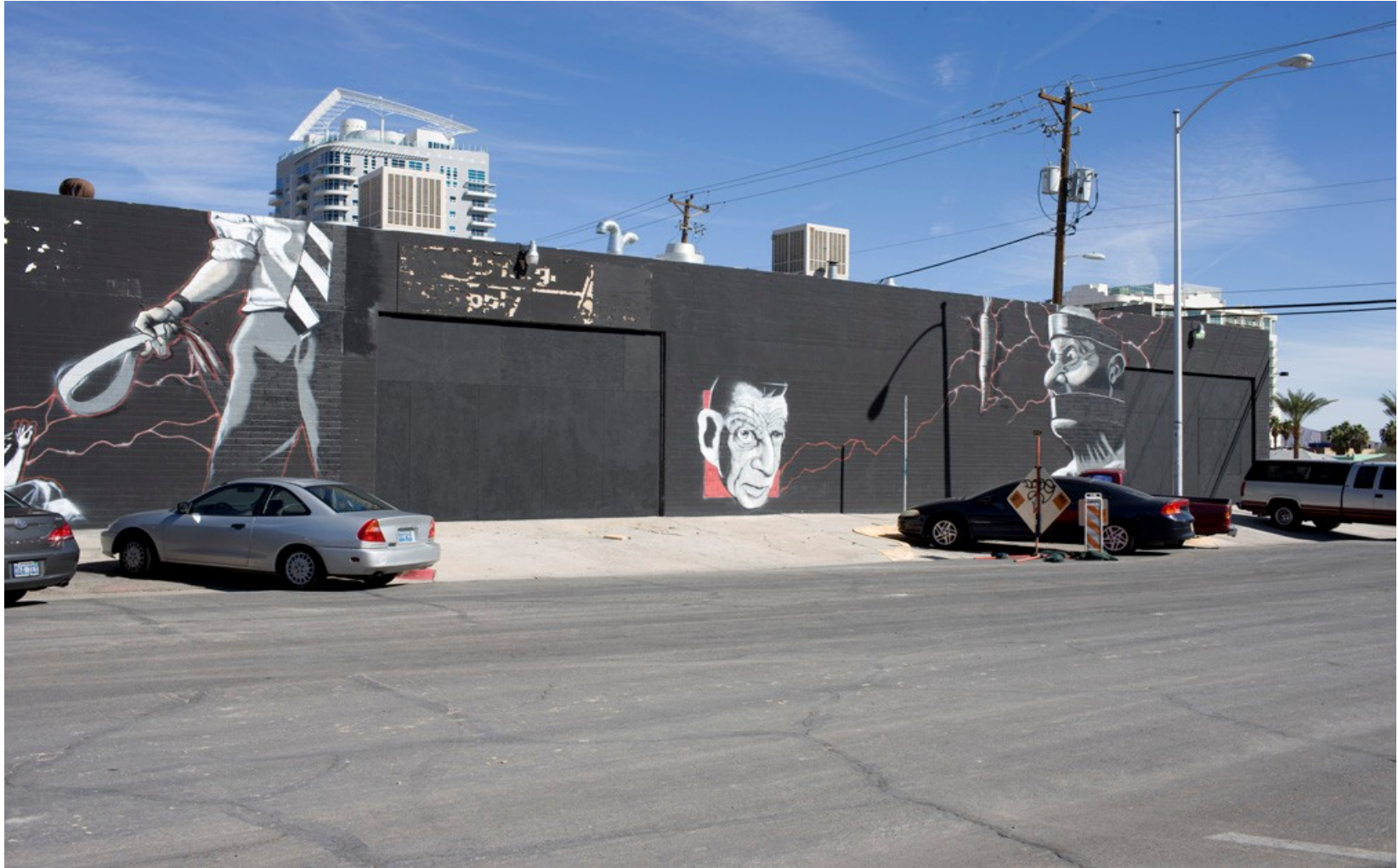
BEFORE PICTURE - 1025 South First Street (Artifice) (South side of the building)
