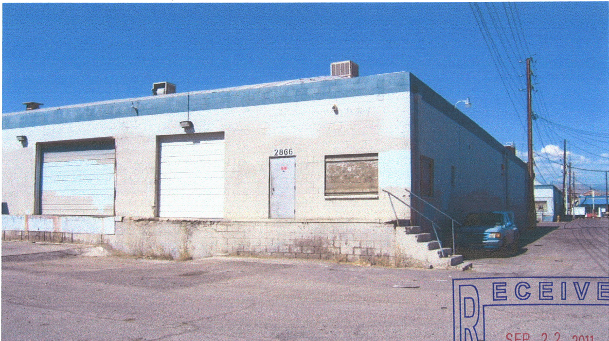
EAST AND NORTH ELEVATIONS
