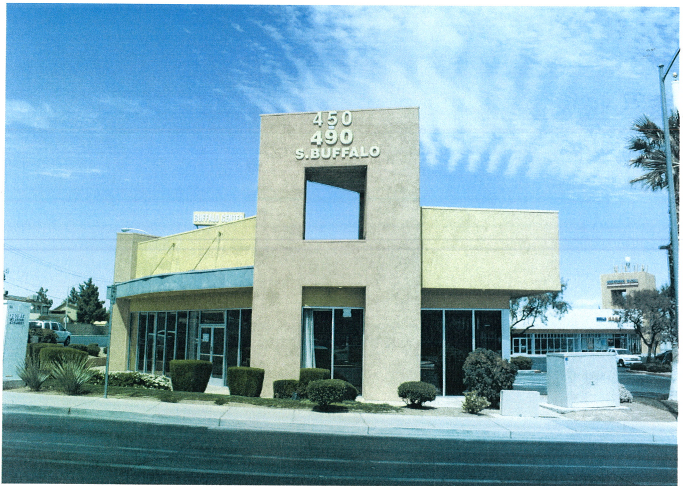
SOUTH FACE OF BLDG.
