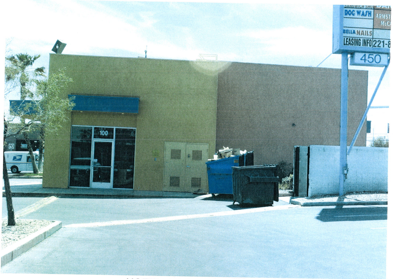
NORTH FACE OF BLDG.
