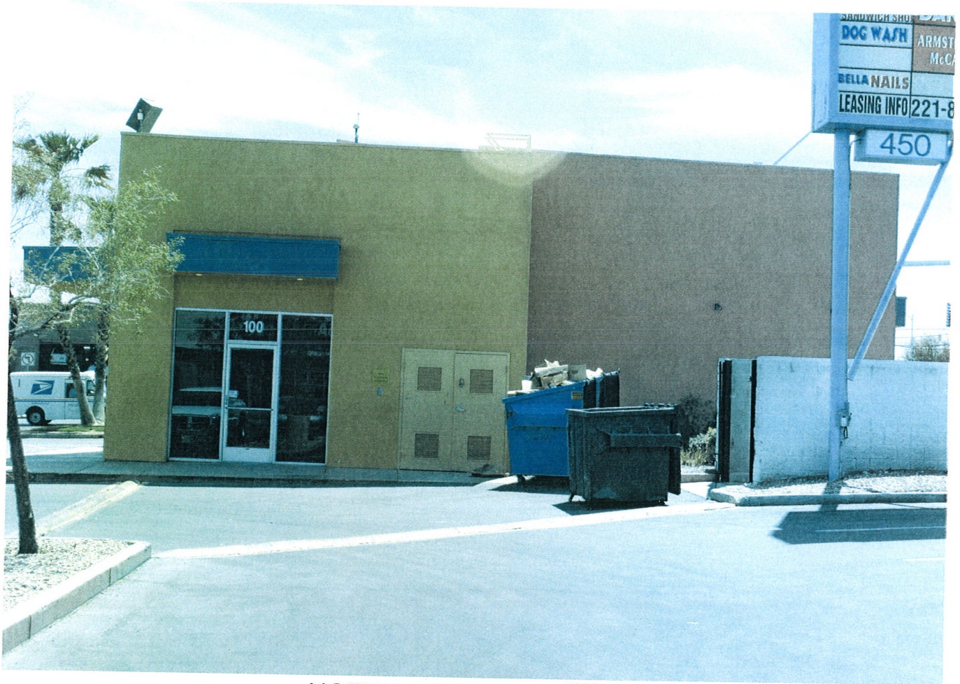
NORTH FACE OF BLDG.
