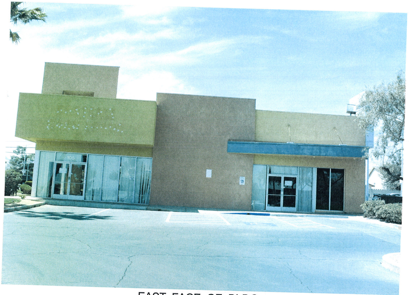
EAST FACE OF BLDG.
