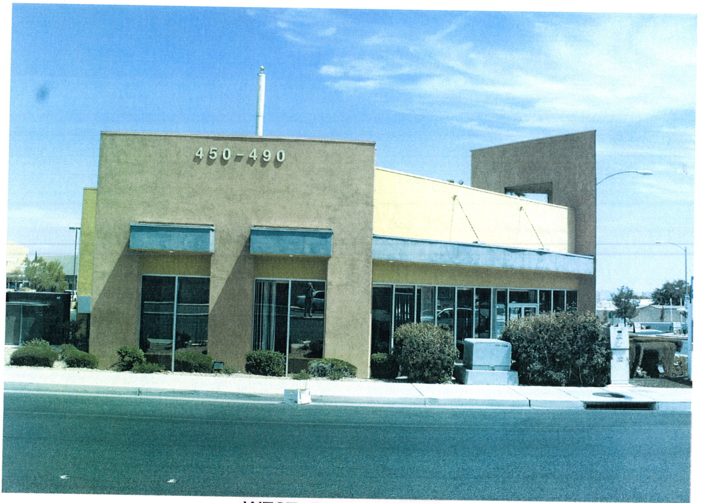
WEST FACE OF BLDG.
