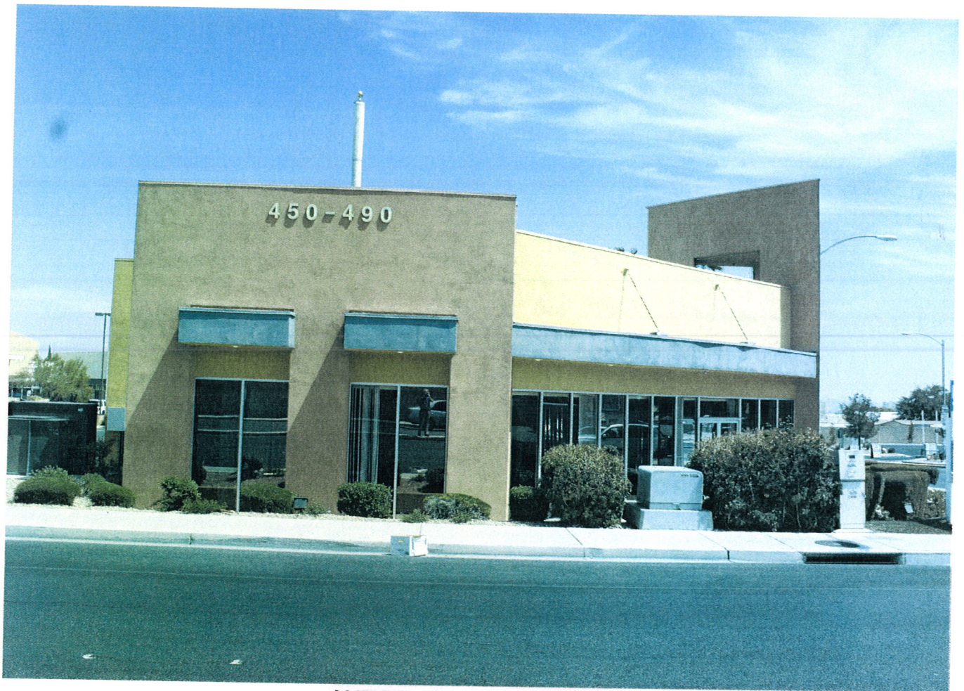
WEST FACE OF BLDG.
